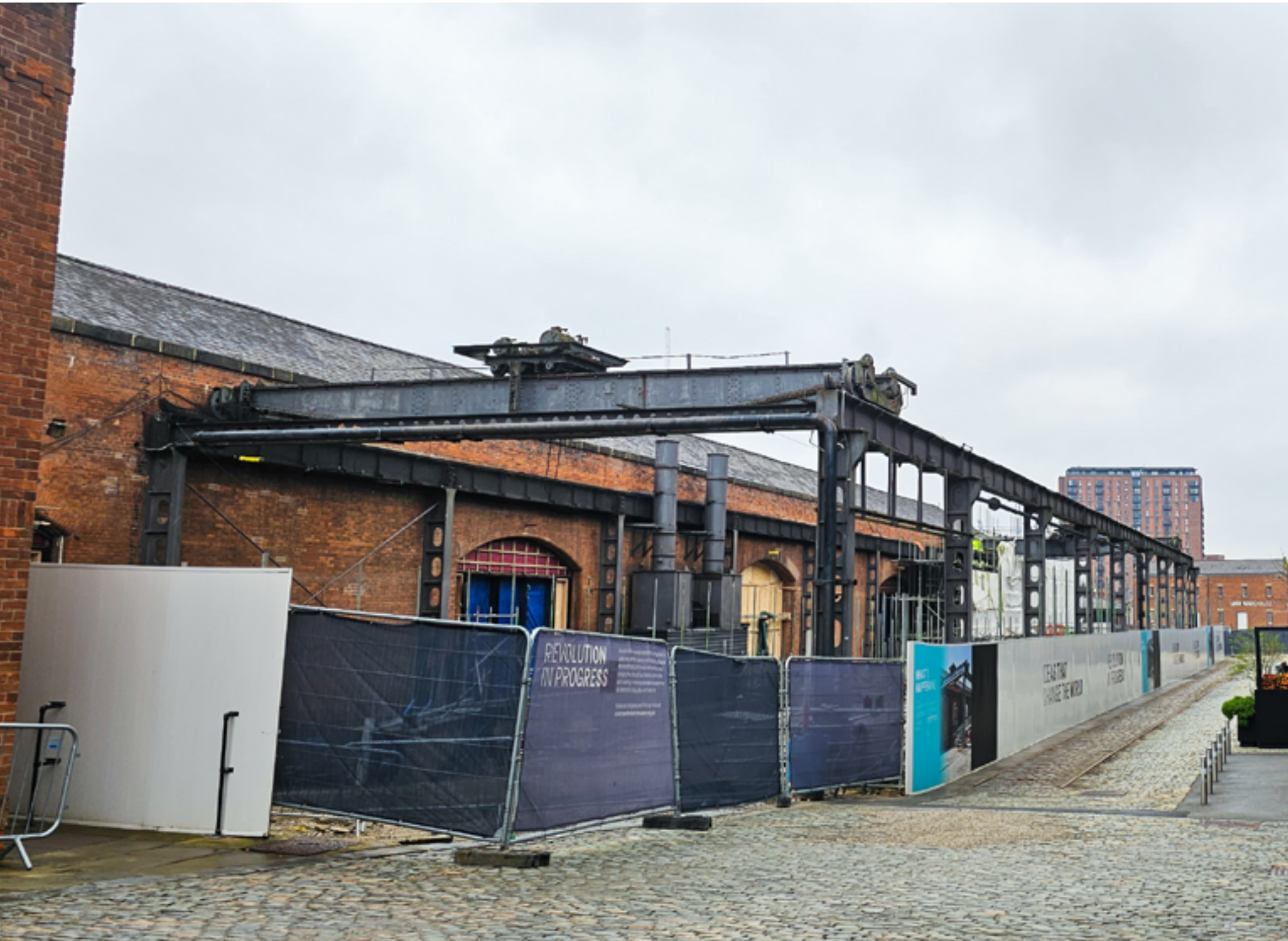
Figure 4 Power Hall North Elevation showing the Gantry Crane
