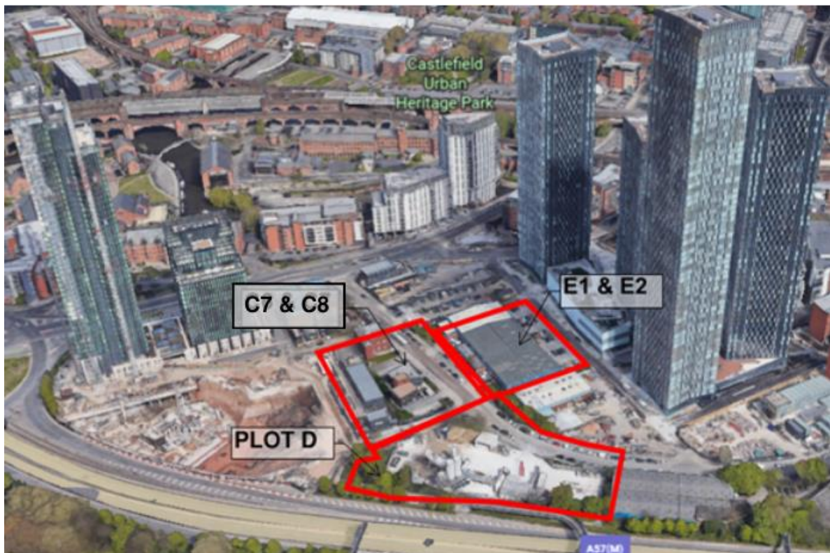
Figure 1 - Google Earth image of the Site Location, 2022
