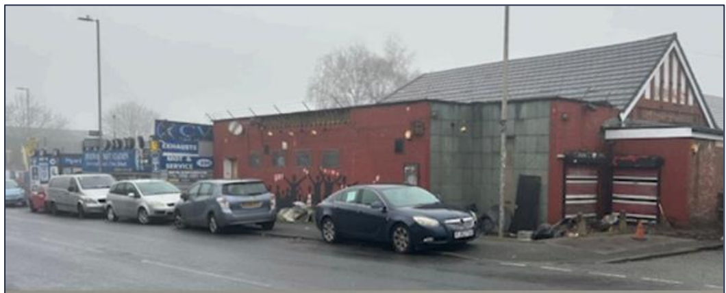
Figure 2.1 – View of Site from Moston Lane
