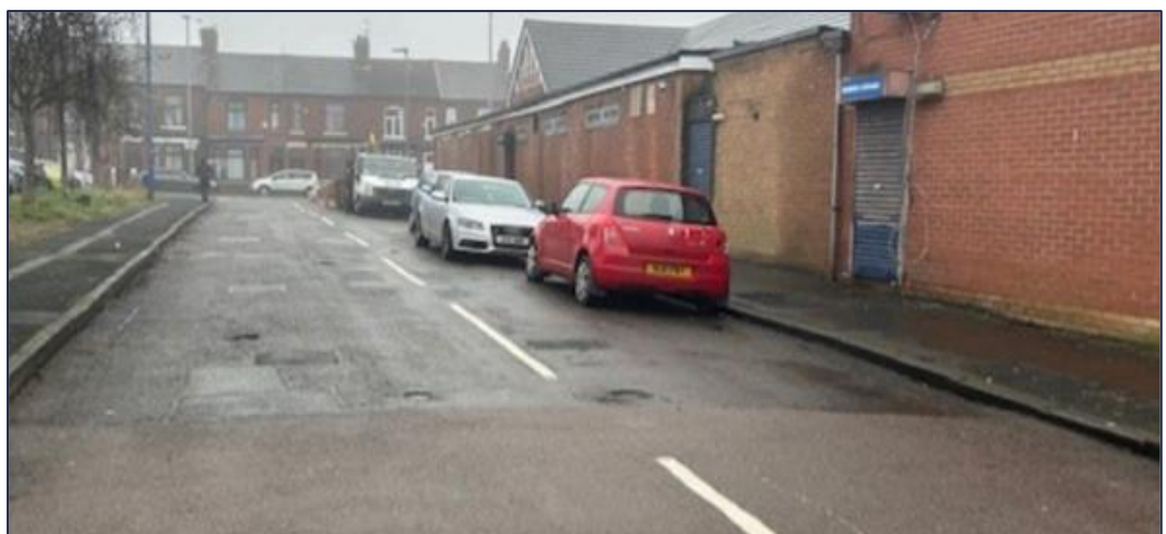
Figure 2.2 – View of Site from Penn Street
