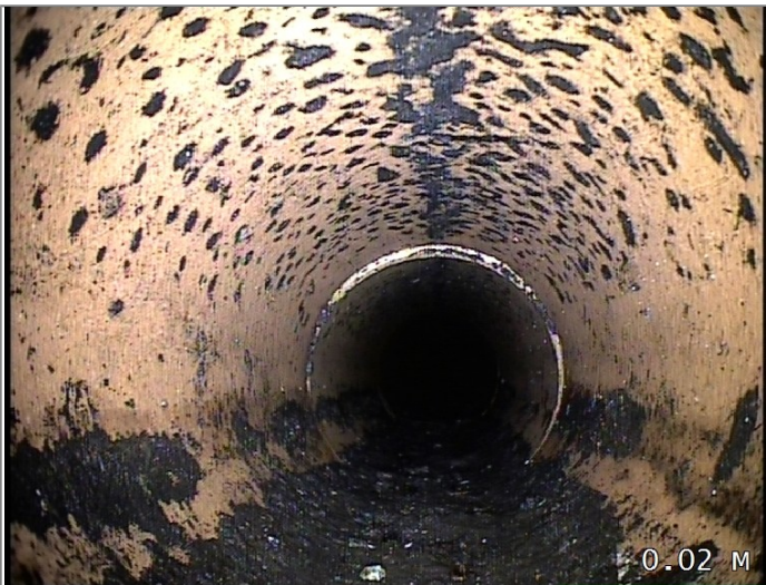
Start node type, manhole, reference MH 03
