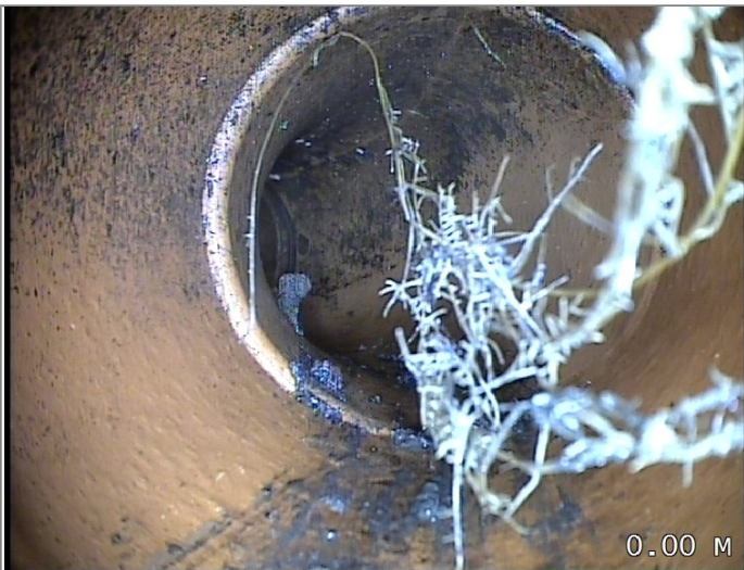
Start node type, manhole, reference MH 02
