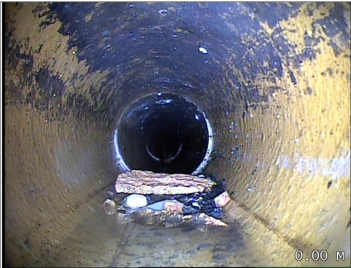
Start node type, manhole, reference MH 02
