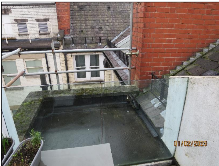
PHOTO 06 – Small flat roof from flat 401 balcony
