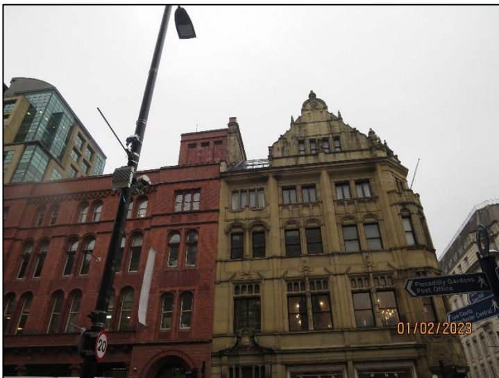
PHOTO 03 – External, King Street façade
