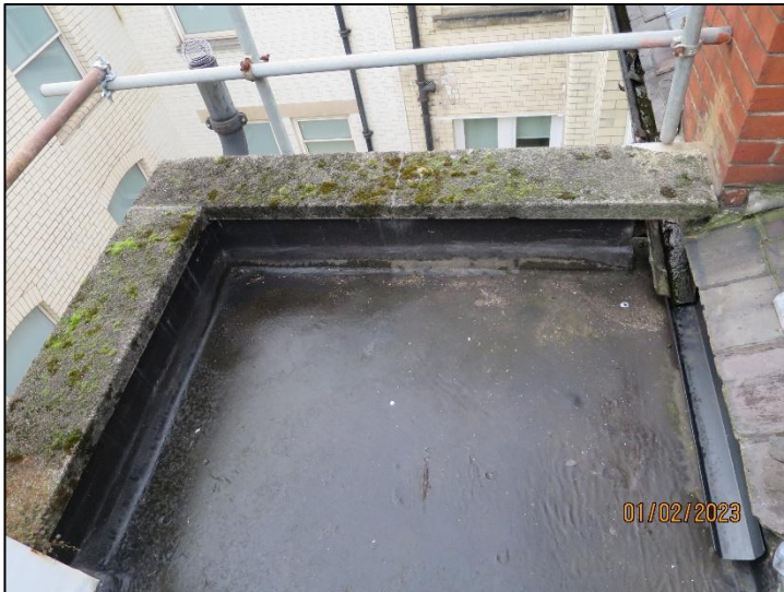
PHOTO 05 – Small rear lightwell elevation flat roof at high-level
