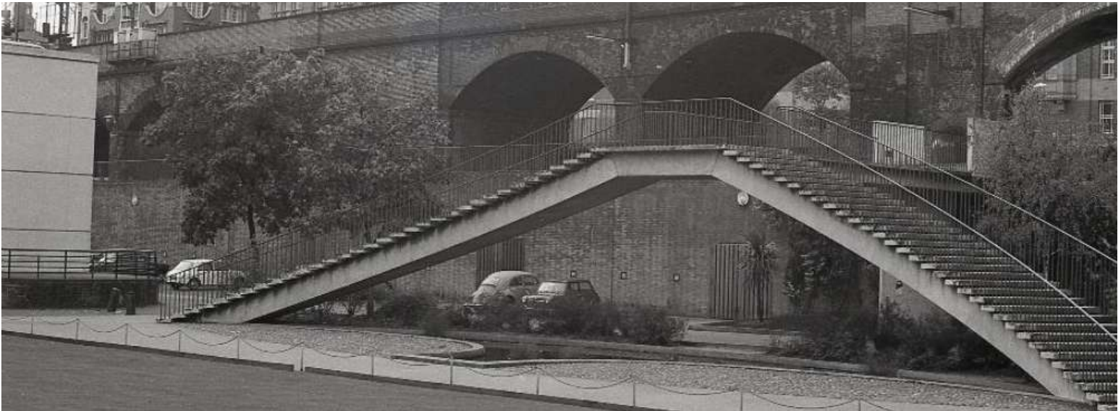
Newly completed butterfly stair, 1962. Photo: SLHA, ID Manchester, pp. 170
