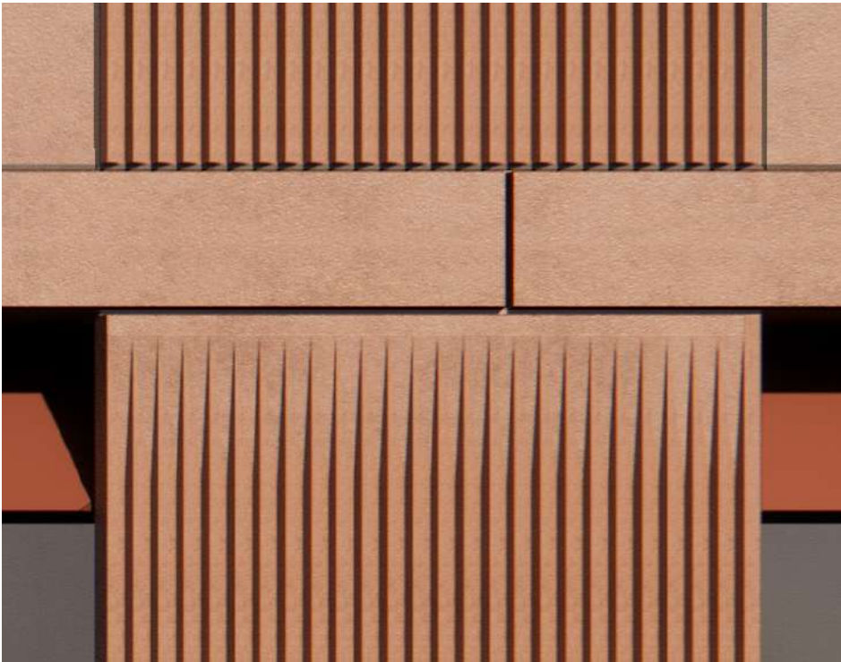
Feathered detail at top of profiled east and west piers
