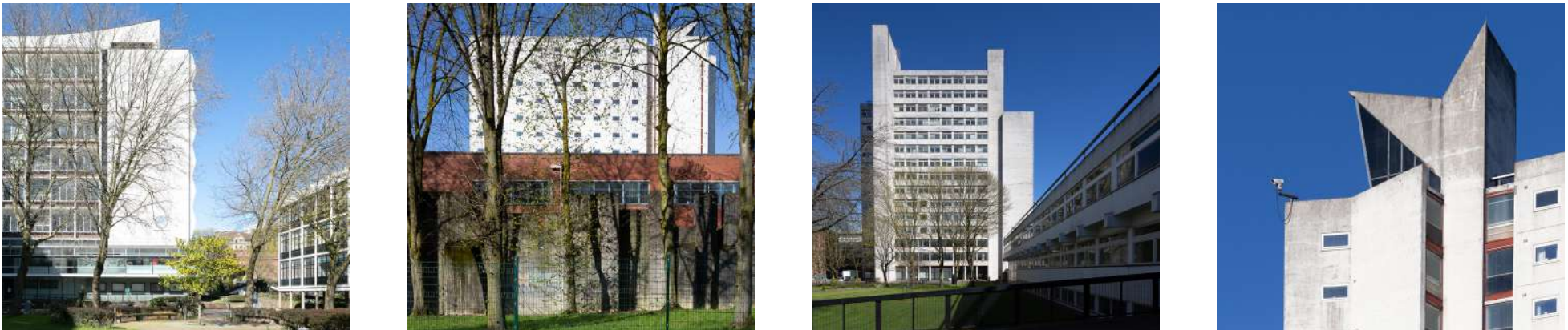
Former campus Modernist buildings and structures
