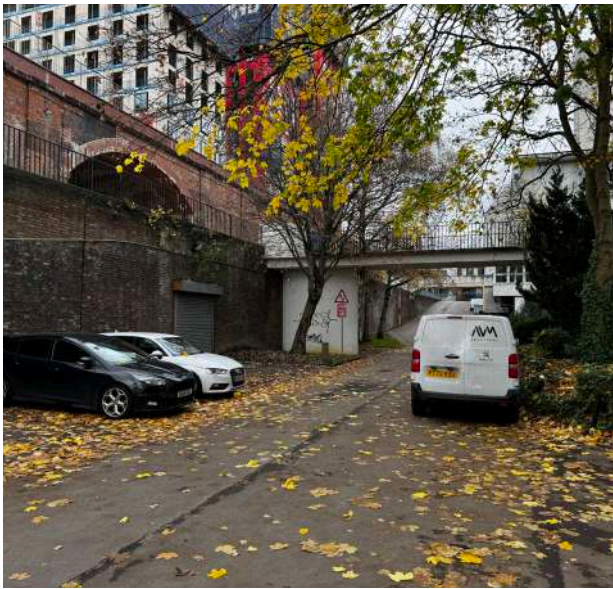
Lower Altrincham Street An open air service road currently facilitates servicing of the buildings immediately south of Altrincham Street. The Butterfly Stairs span over the road, managing the separation of pedestrians from the heavy goods vehicles and cars that regularly use this route. The road is on-show to people enjoying the adjacent Bowling Green.
