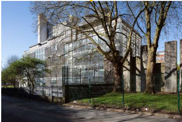
Morton Laboratory, Holloway Wall and retaining walls to London Road verge
