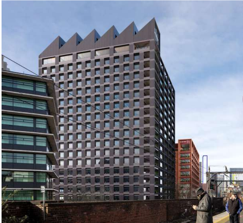
East elevation from Platform 14 [Our Studio]
