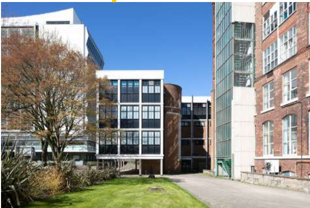
Renold Building, Manchester Meeting Place and the Mill on approach from the south
