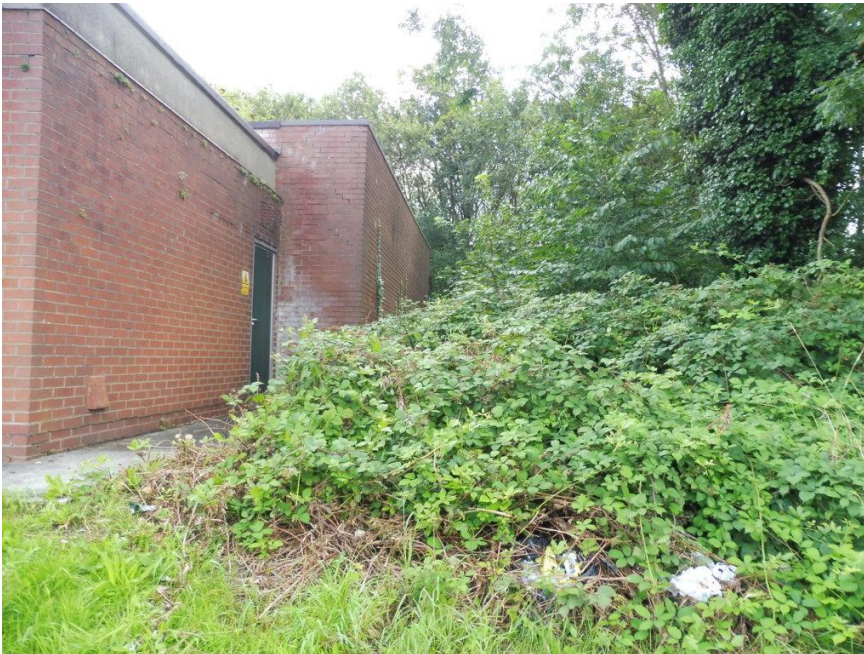
Photograph 12: View of large utility building whose location cuts into the western margin of the site (see also Figure B aerial image for location of structure)
