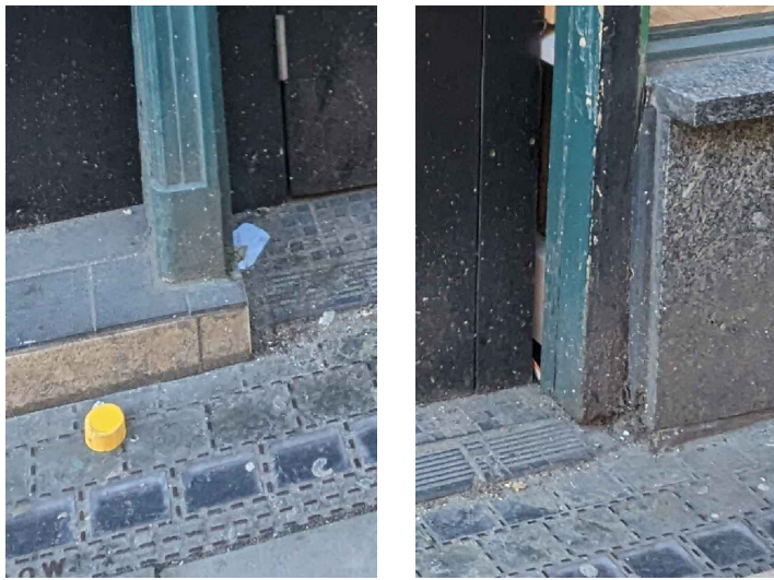
EXISTING ENTRY THRESHOLD
