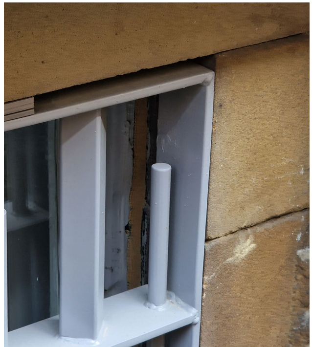
Figure 2 Photograph showing painted fixing to side plates, positioned to rear of bars
