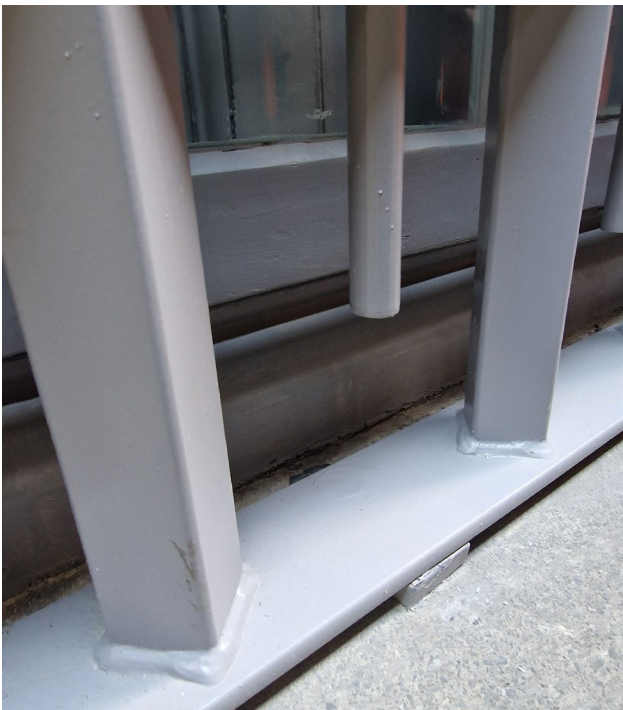
Figure 1 Photograph showing painted fixing to lower plate
