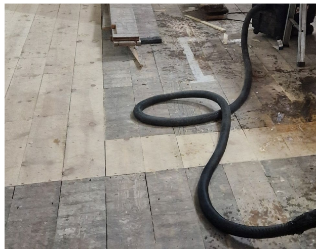
Figure 1 Example spliced boards in-situ
