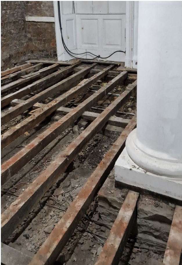
B02-B2-001 Boards Lifted
