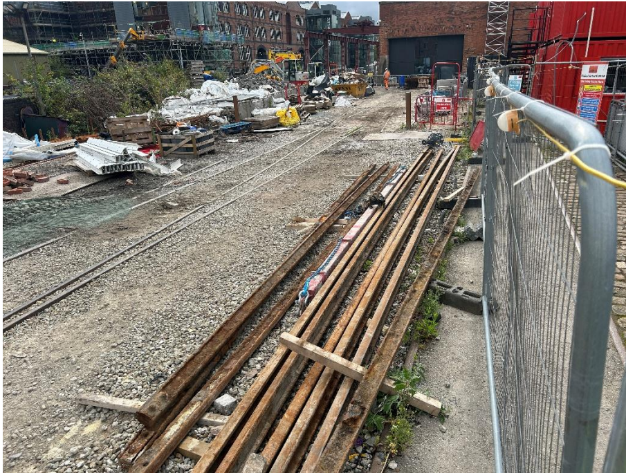
Figure 11 – Ballast Fill Between Tracks
