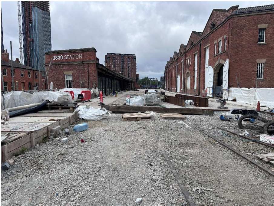
Figure 08 – View from Goods Office Yard – looking West towards 1830 Warehouse & Station Building
