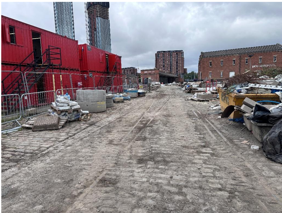
Figure 03 – Cobbles / Setts
