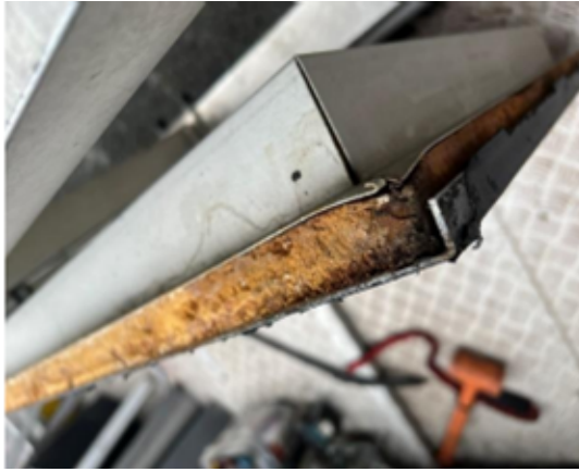
Investigative photographs of spandrel panelling demonstrating extensive water ingress
