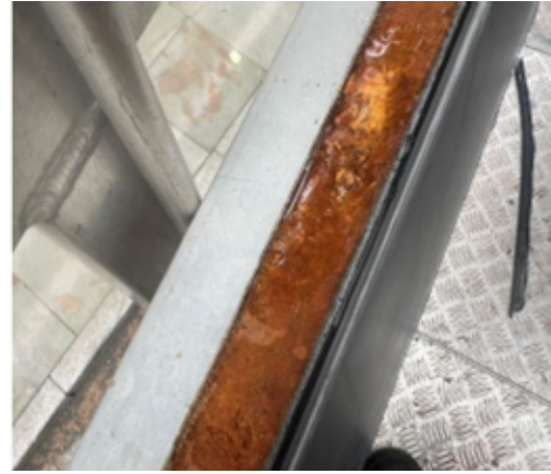
Investigative photographs of spandrel panelling demonstrating extensive water ingress
