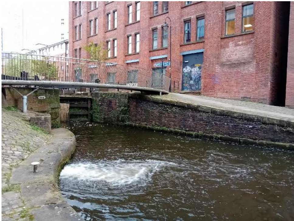
Figure 14: View of sandstone capstones above fired bricks and overflow outlet.
