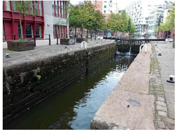
View northeast towards Rochdale Canal Lock Number 89 (Tib Lock) and modern office block located on the site of former Havelock Mills.
