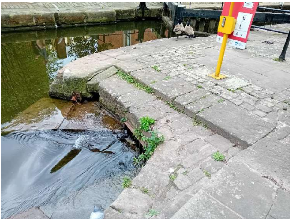
Figure 15: View of overflow inlet to the northeast of the lock
