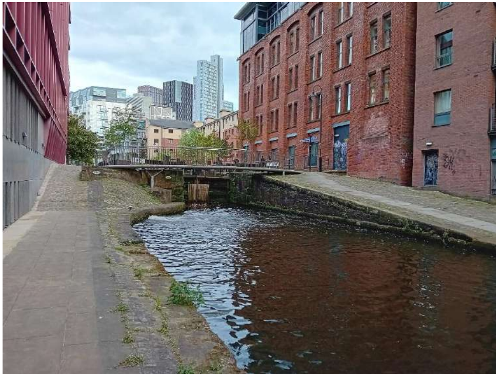
Figure 12: View of Millenium Bridge that spans the Rochdale Canal
