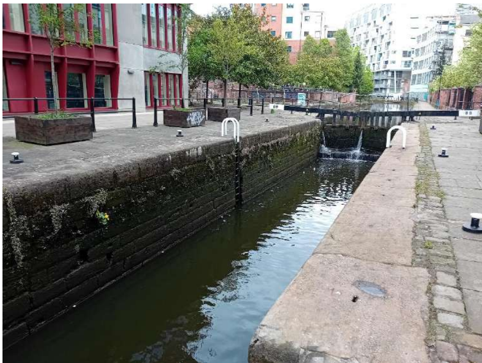
Figure 13: View of sandstone blocks within the lock chamber
