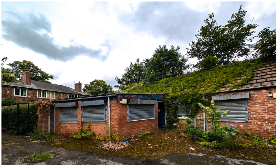
3. Building to be Demolished
