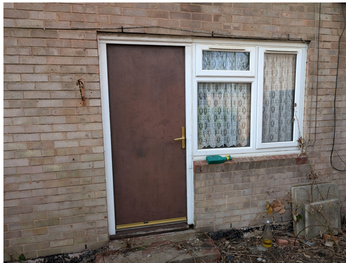
Image Two: Existing Back Door and Window to Lounge
