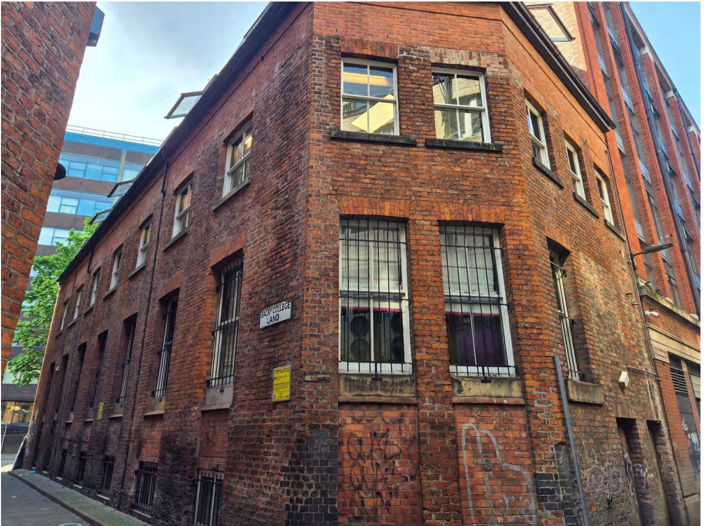
Plate 16 View showing the southern elevation of 5 The Parsonage, with basement level visible along Back College Land, facing north-west
