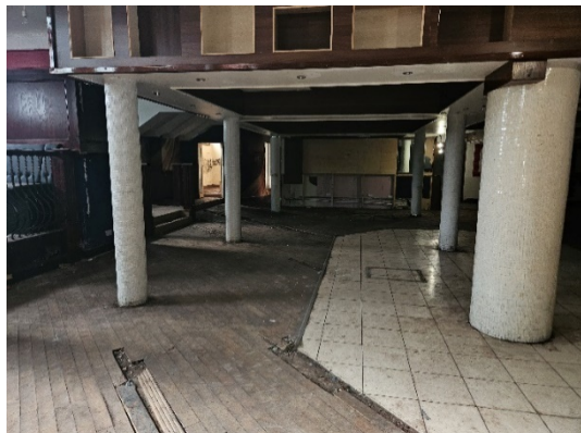
Photograph 9: Ground level of basement level
