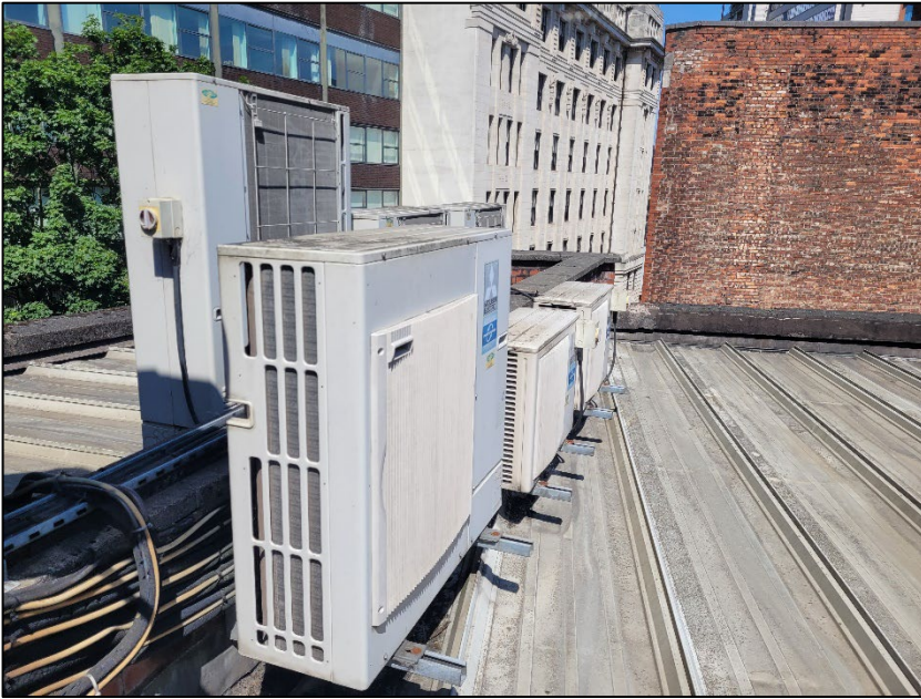
Photograph 4 Southern structure at roof level
