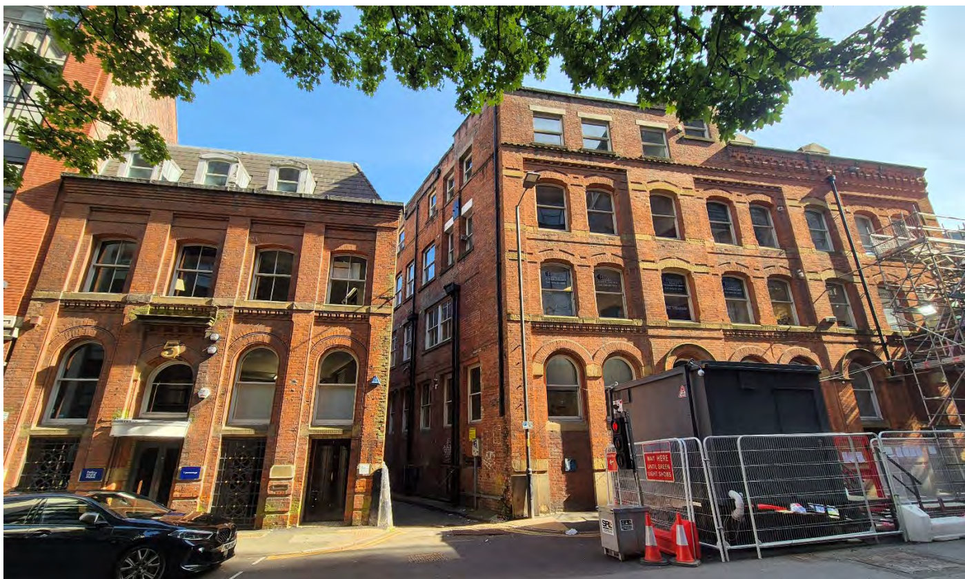
Plate 14 View showing the western elevation of 1 North Parade and 5 The Parsonage
