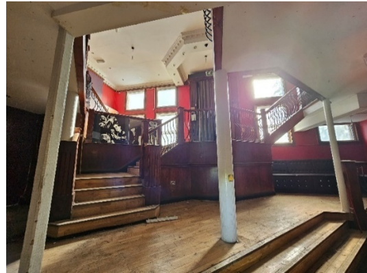
Photograph 8: Upper floor access from inside basement level
