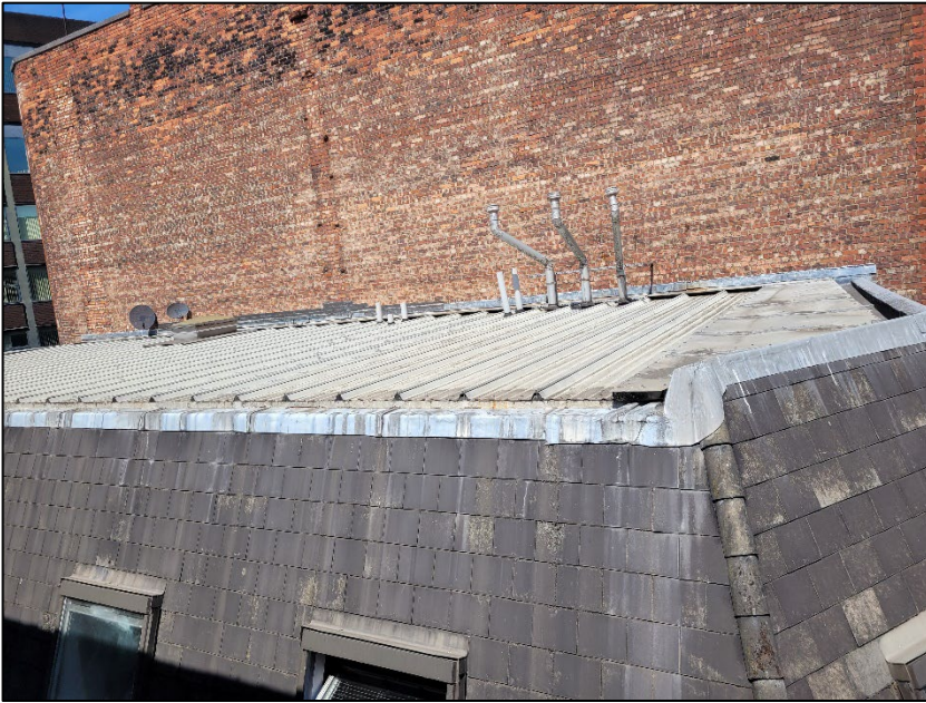
Photograph 7 Roof of northern building and parti wall with the joining structure to the north
