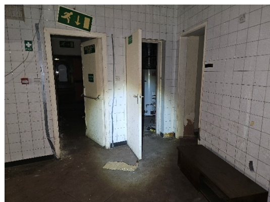
Photograph 12: Boiler room and fire exit ahead
