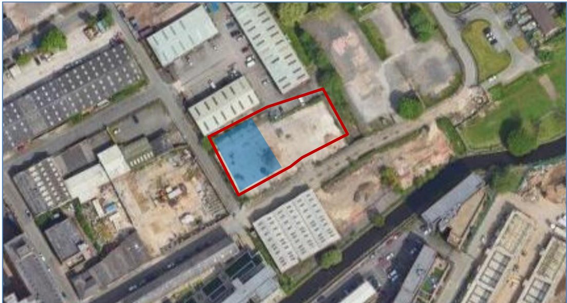
Plate 1: Recent aerial view of Eliza Yard prior to redevelopment with the excavation area highlighted blue
