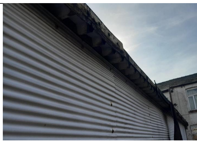
Photo 11: West view of the shed on-site, comprised of metal panels and a corrugated bitumen roof.
