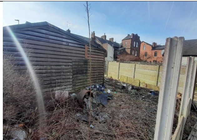
Photo 1: North view of the shed on-site, comprised of metal panels and a corrugated bitumen roof.
