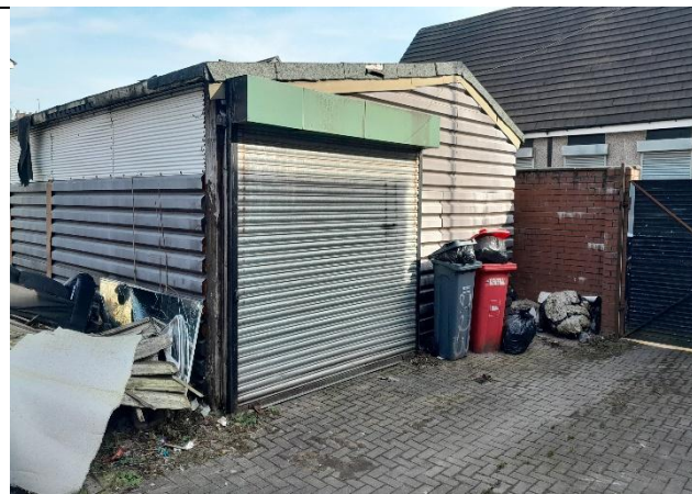
Photo 5: South view of the shed on-site, comprised of corrugated metal panels and a bitumen roof.
