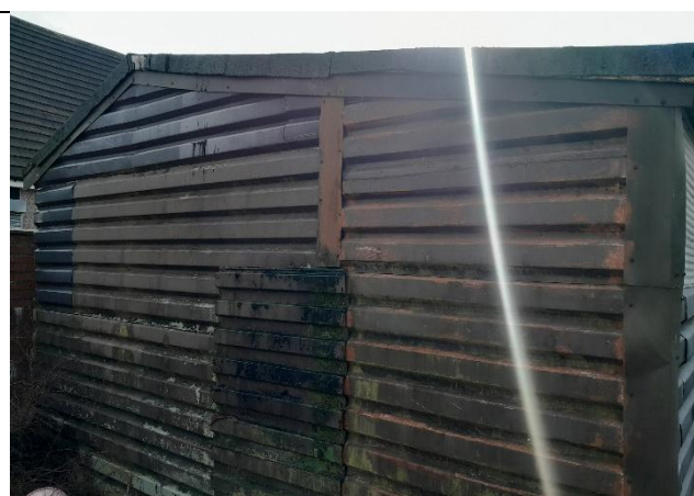
Photo 12: North view of the shed on-site, comprised of metal panels and a corrugated bitumen roof.
