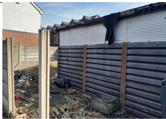
Photo 10: West view of the shed on-site, comprised of metal panels and a corrugated bitumen roof.
