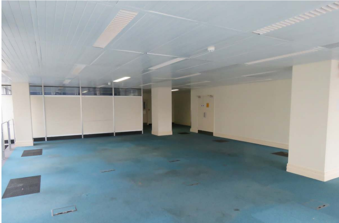
01-10 Looking north-east towards the inserted offices, showing the raised access floor. Skirtings to the columns and handrails are non-original. Floor approximately 300mm above original level.
