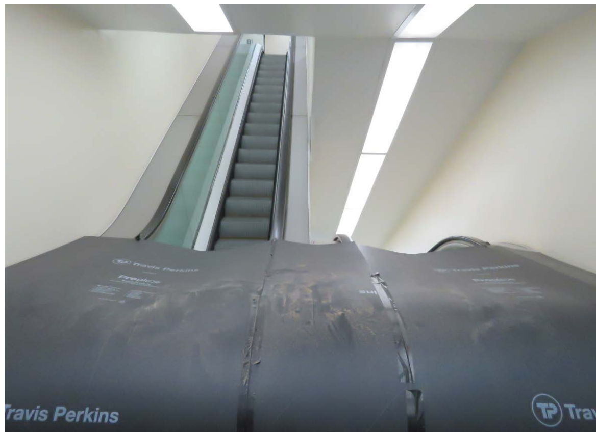
01-22 The currently decommissioned escalators, looking south.
