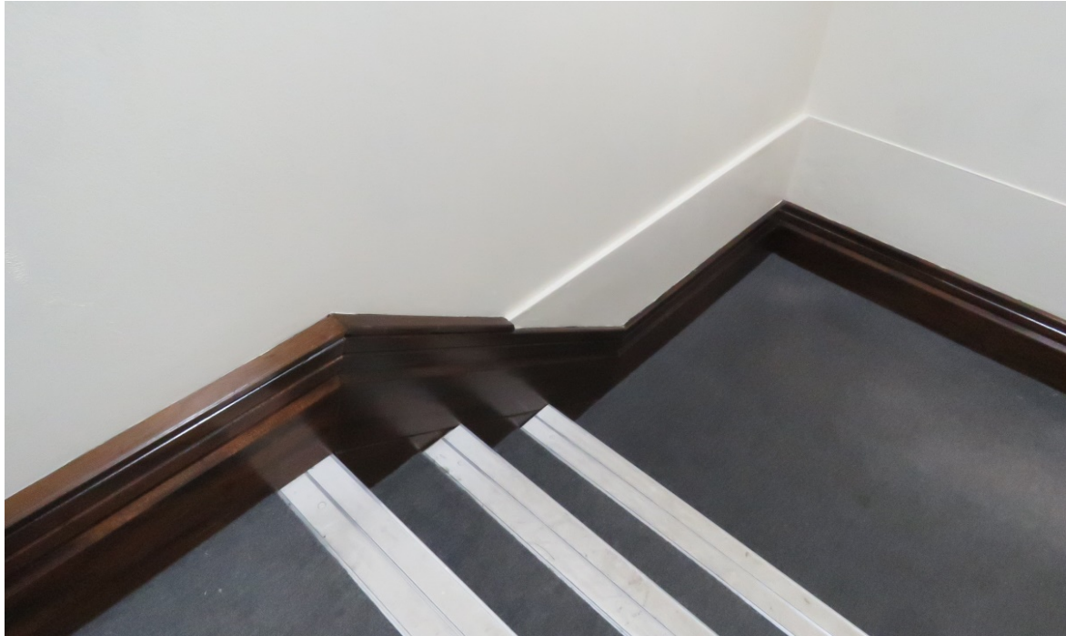
01-14 Detail of surviving skirting in the added stair lobby south-east stair lobby. The fire lobby was added as an extension to the corridor and to accommodate the raised access floor.
