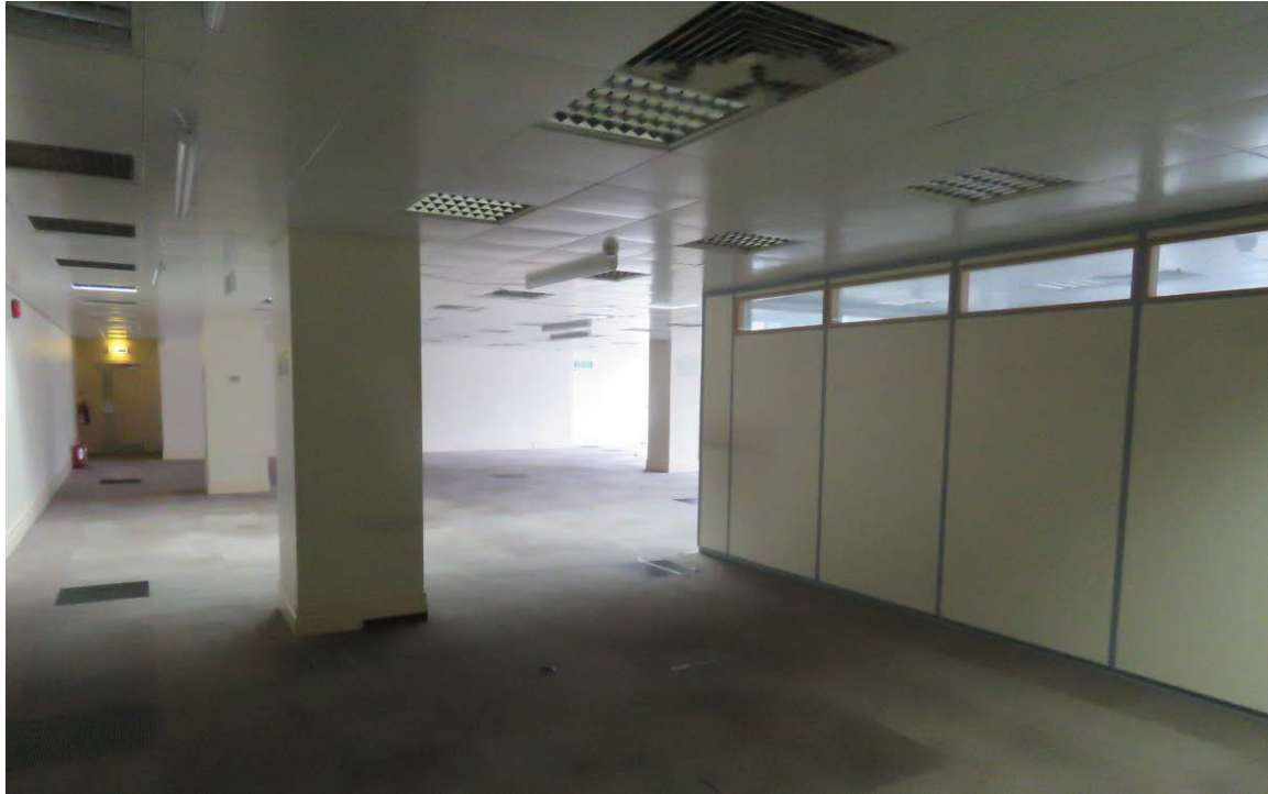
01-12 Looking east across the podium floor, showing the inserted offices.
