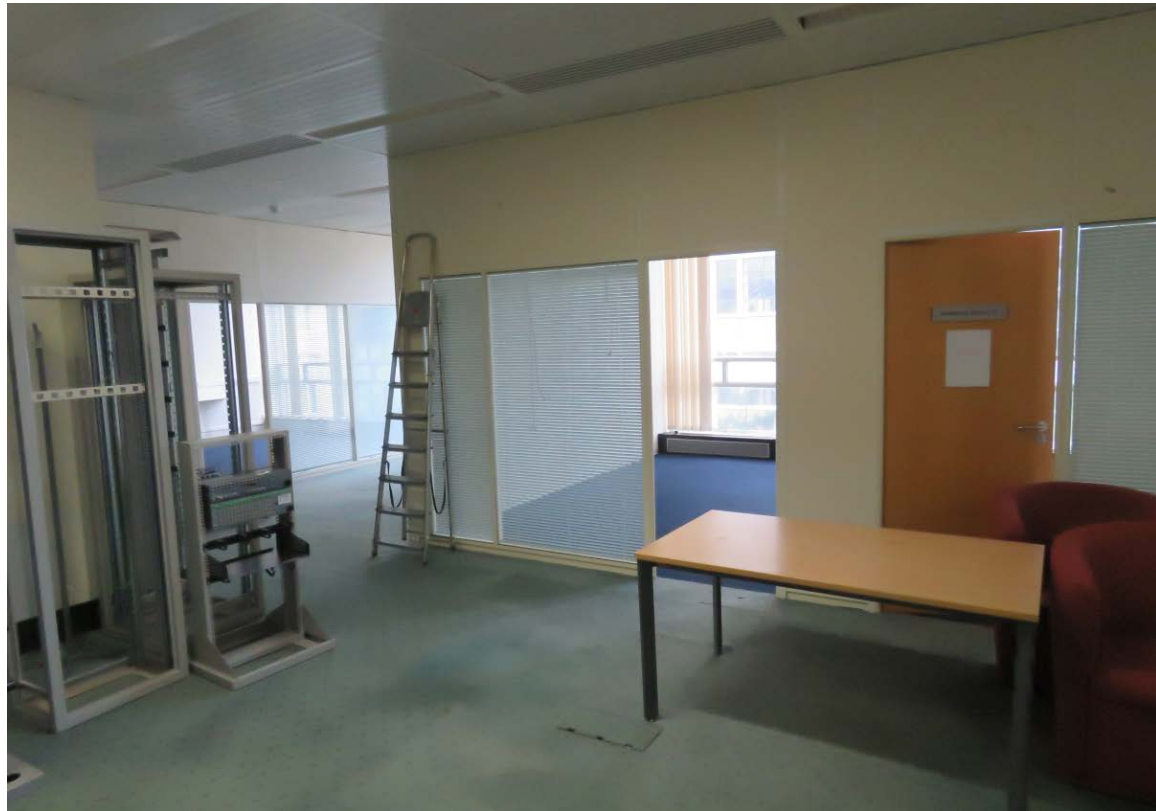
01-06 Looking south-west toward the inserted offices enclosing the Dantzig Street frontage.
