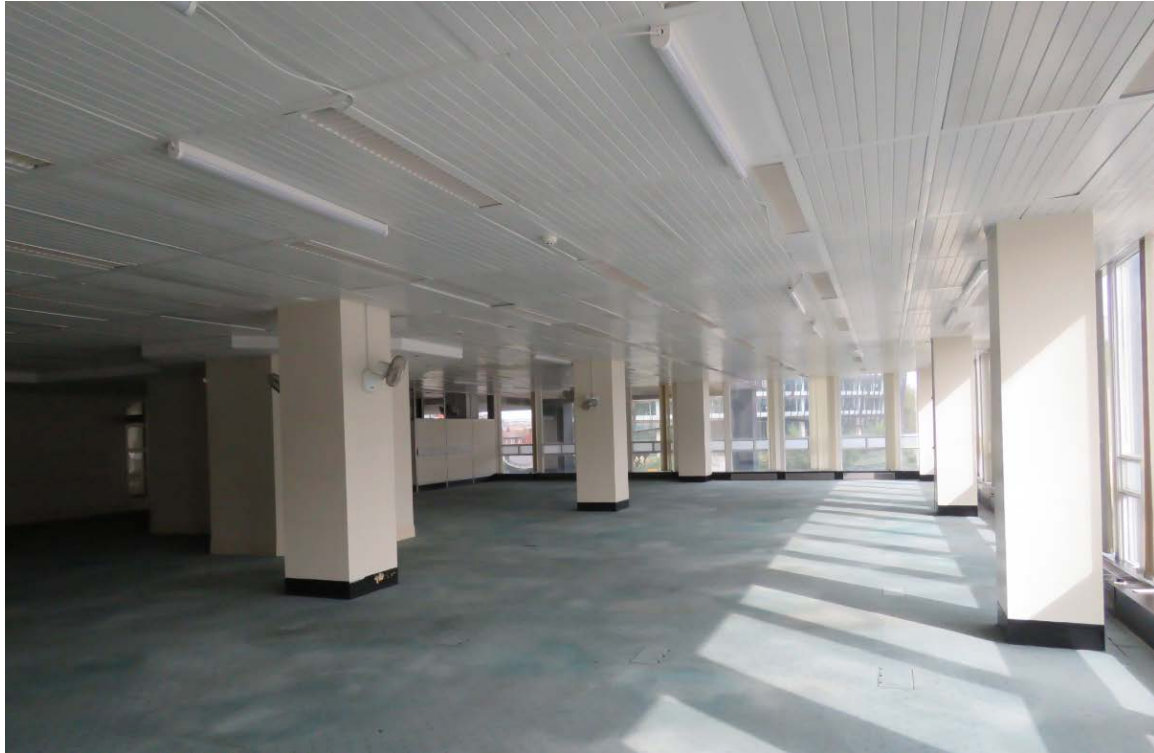
01-18 Looking north towards the portico across the tower office floor. Note the increased proportions as the floor level is at the original level.
