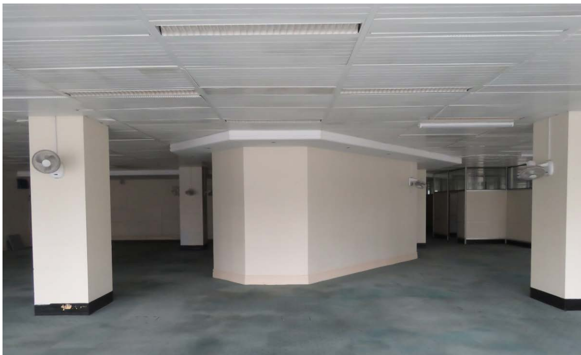
01-19 Looking west across the tower office toward the inserted enclosure of the north-east escape stairs.
