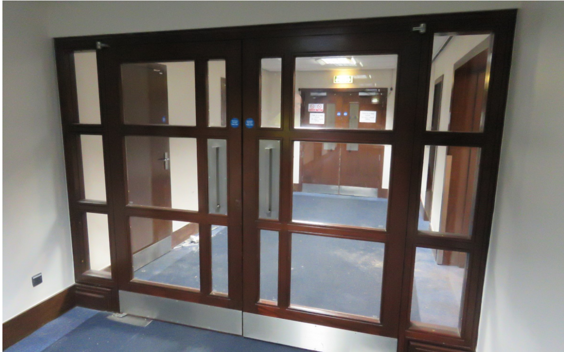
01-02 Looking north through the inserted fire lobby door toward the tower office entrance.
