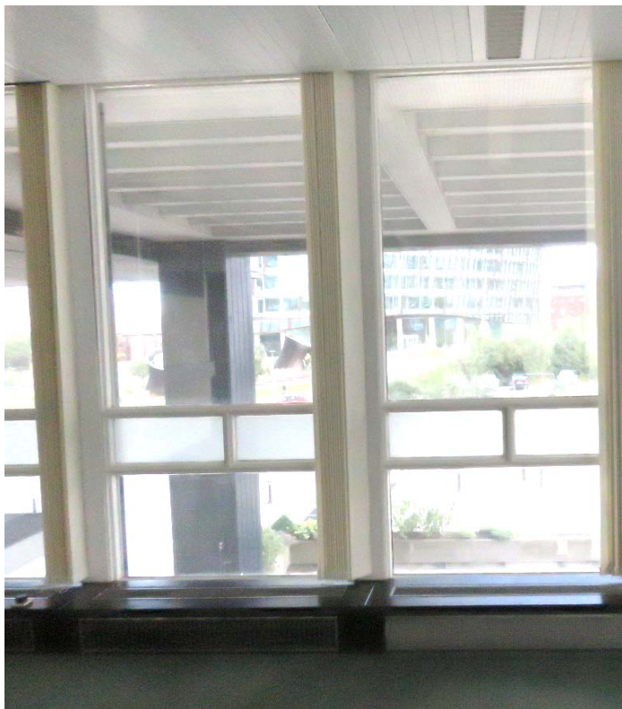
01-21a and 01-21b Looking north from the tower office showing the perimeter Weathermaster, the fenestration pattern (painted white) and the exposed concrete of the portico's soffit.
