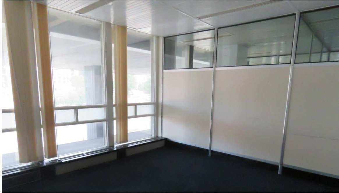
01-04 Looking north-east at the surviving original office partitions and the portico.
