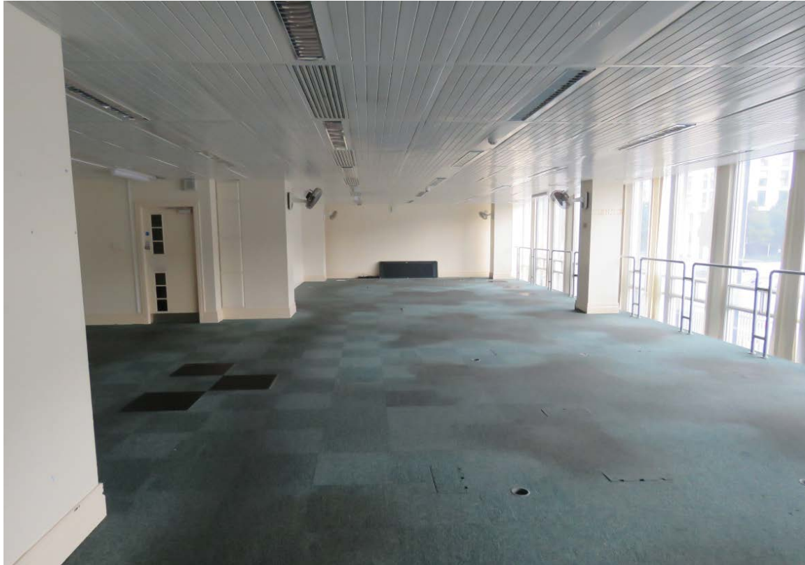
01-16 Looking north across the raised access floor of the enclosed office. Handrails and partitions are non-original, as is the raised access floor.
