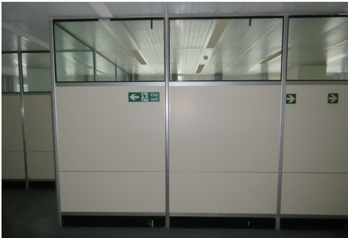
01-03 Looking north from the office entrance at the original partitions which enclose the offices under the portico.
