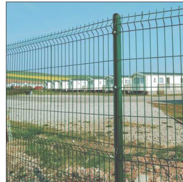
Indicative image of typical site boundary fence
