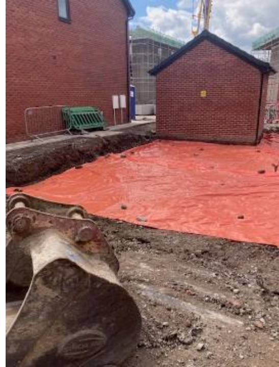
No dig membrane being installed to rear gardens of Plots 18/19
