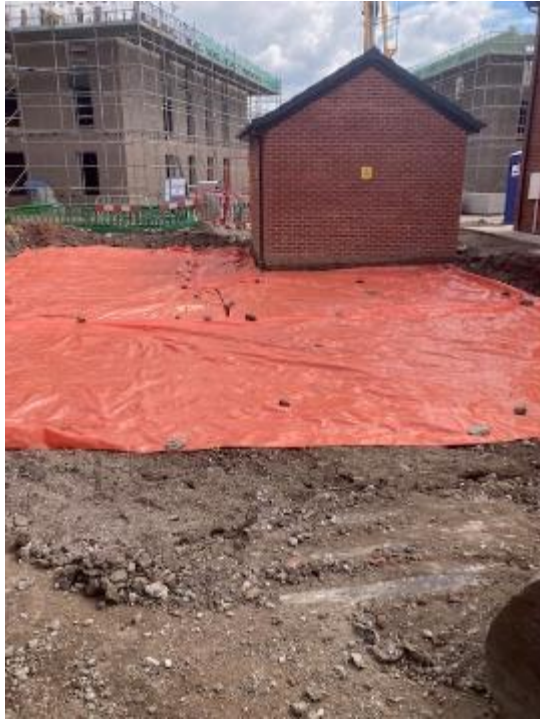
No dig membrane being installed to rear gardens of Plots 18/19
