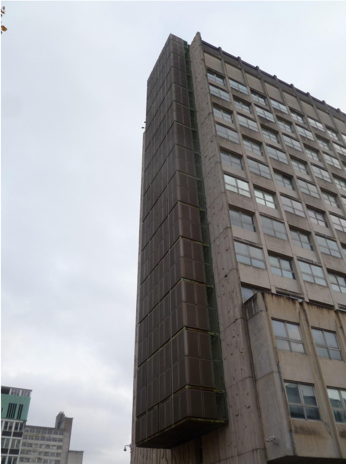
Façade facing Drover Lane showing later addition of metal flue containment.
