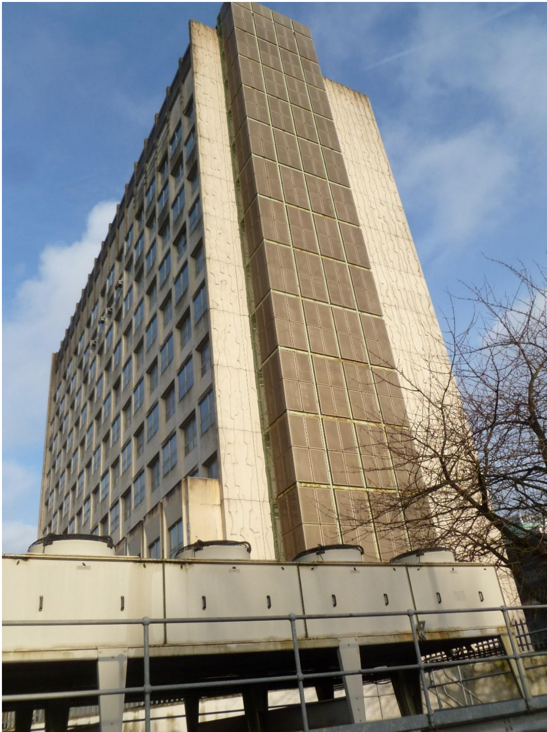
View from Sackville Street looking north showing added flue containment.
