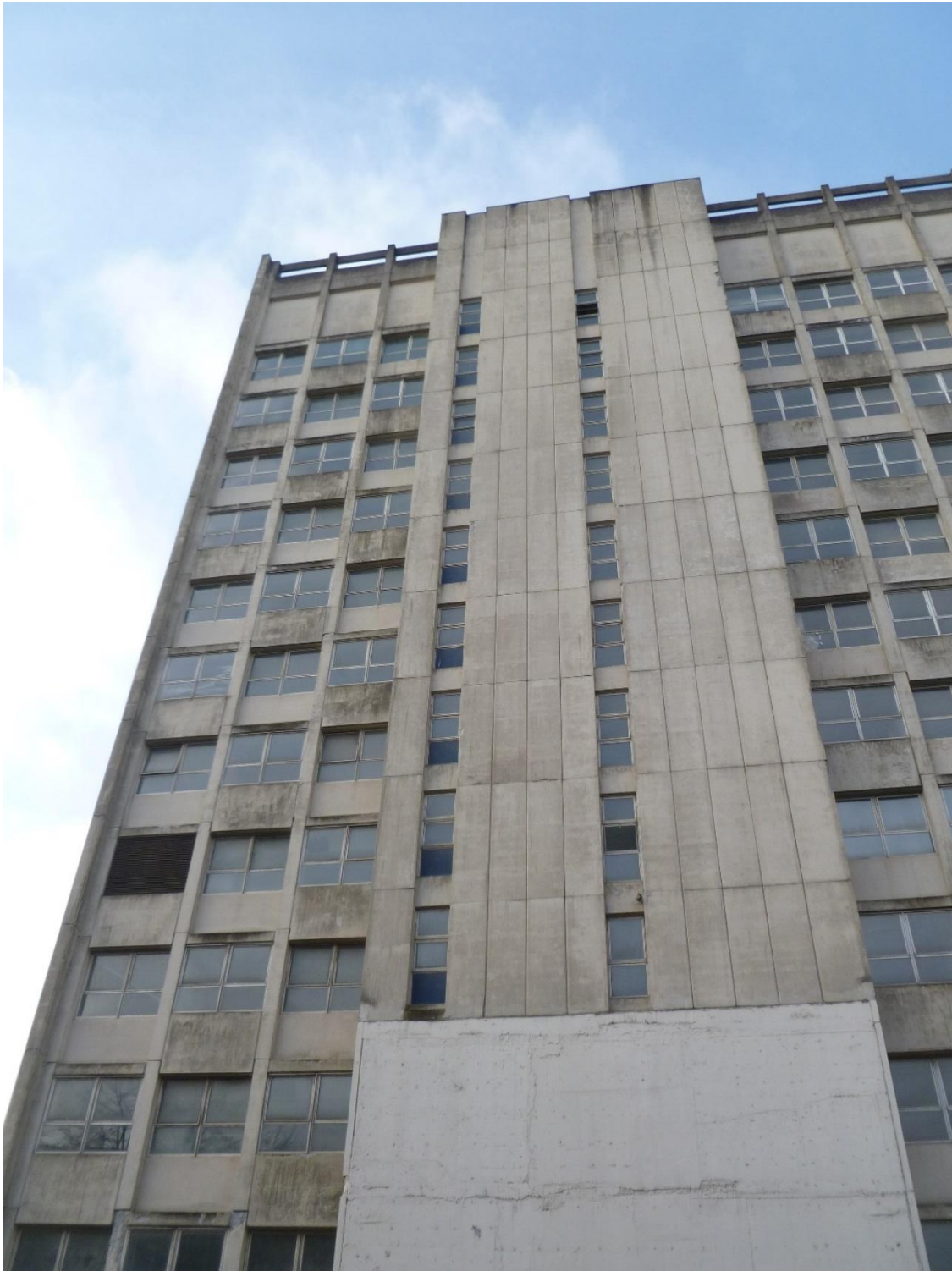
Façade to Sackville Street showing location of removed bridge link and entrance.
