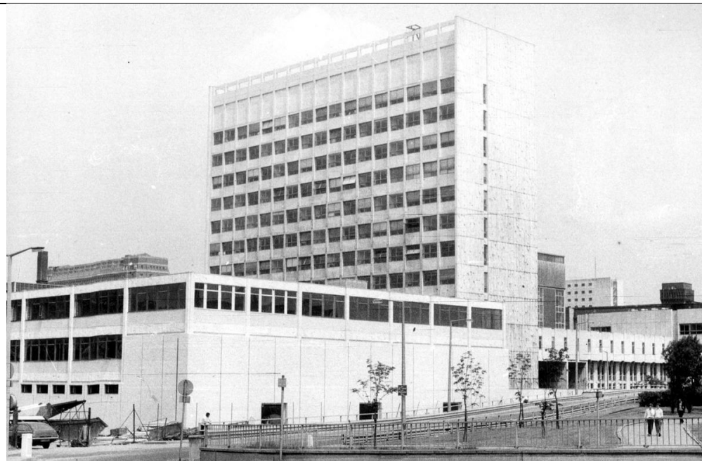
UMIST Chemistry Building, June 1973. Source: MCC Local Image Archive (GM Lives)
