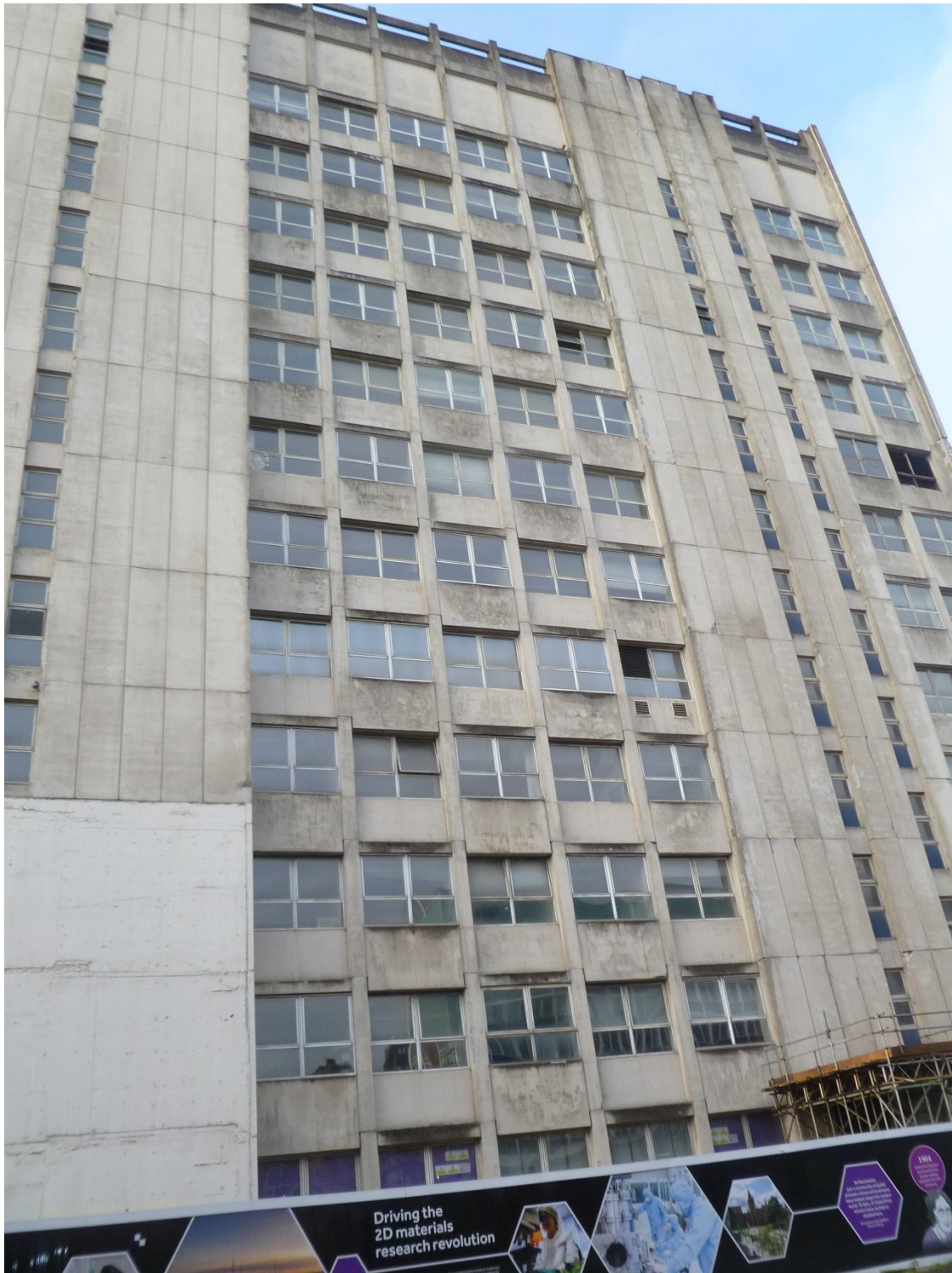
Façade to Sackville Street showing location of removed bridge link and entrance to left of picture.
