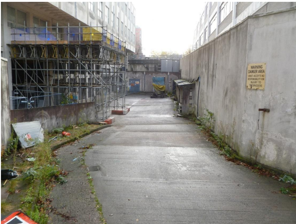
View into service yard from Drover Lane.
