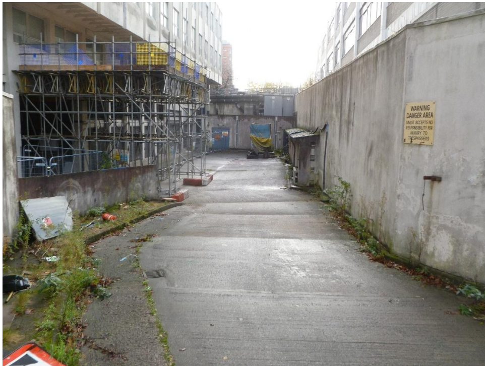
Figure 6.2: Scaffolding constructed to provide safe access into the rear entrance.
