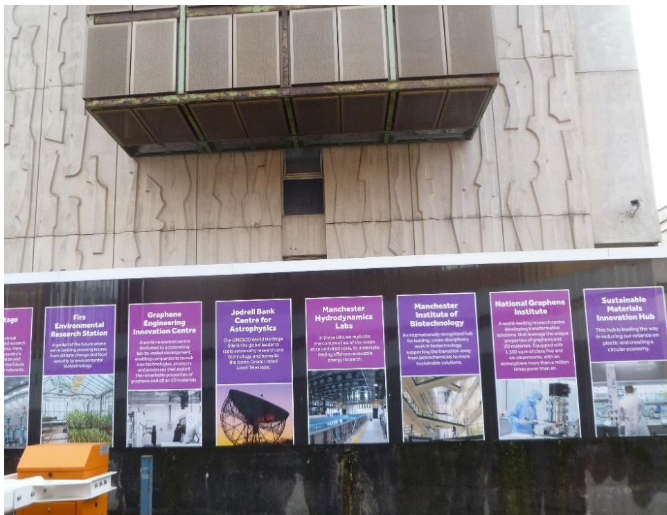
Later flue containments covering and altering original fenestration.
