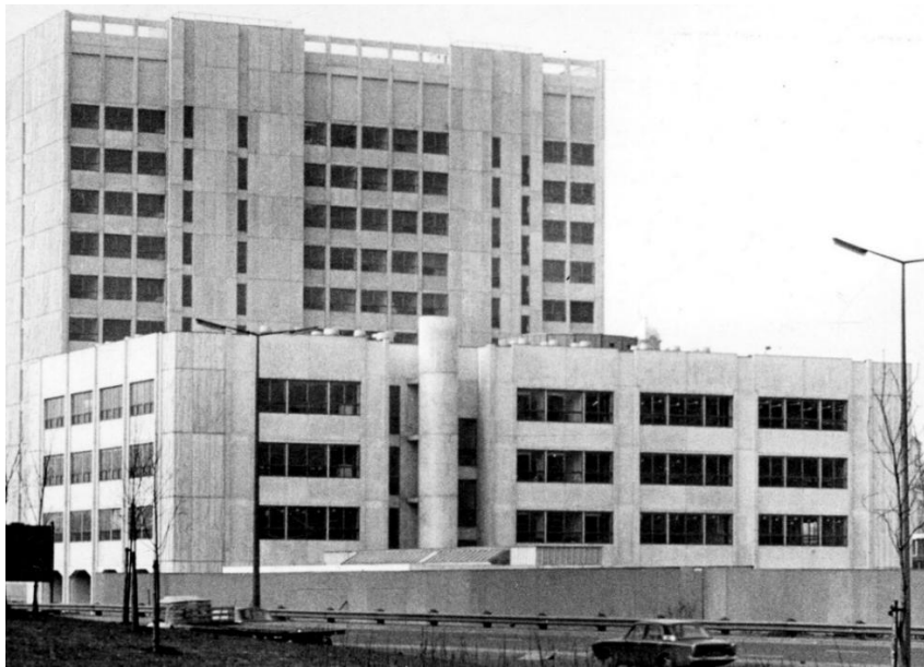
Figure 5.2: View of the Chemistry Building shortly after completion in c.1968 looking west from Mancunian Way. The four storey undergraduate part of the building in the foreground has been demolished.
