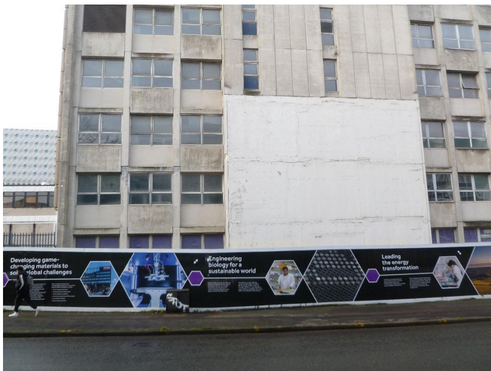
Façade to Sackville Street showing location of removed bridge link and former entrance.
