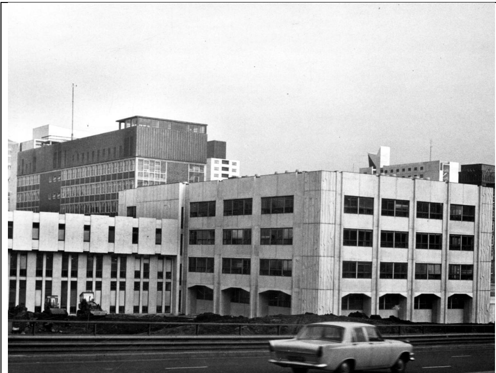
Manchester College of Technology Building from Mancunian Way, Manchester 1968. Source: MCC Local Image Archive (GM Lives)
