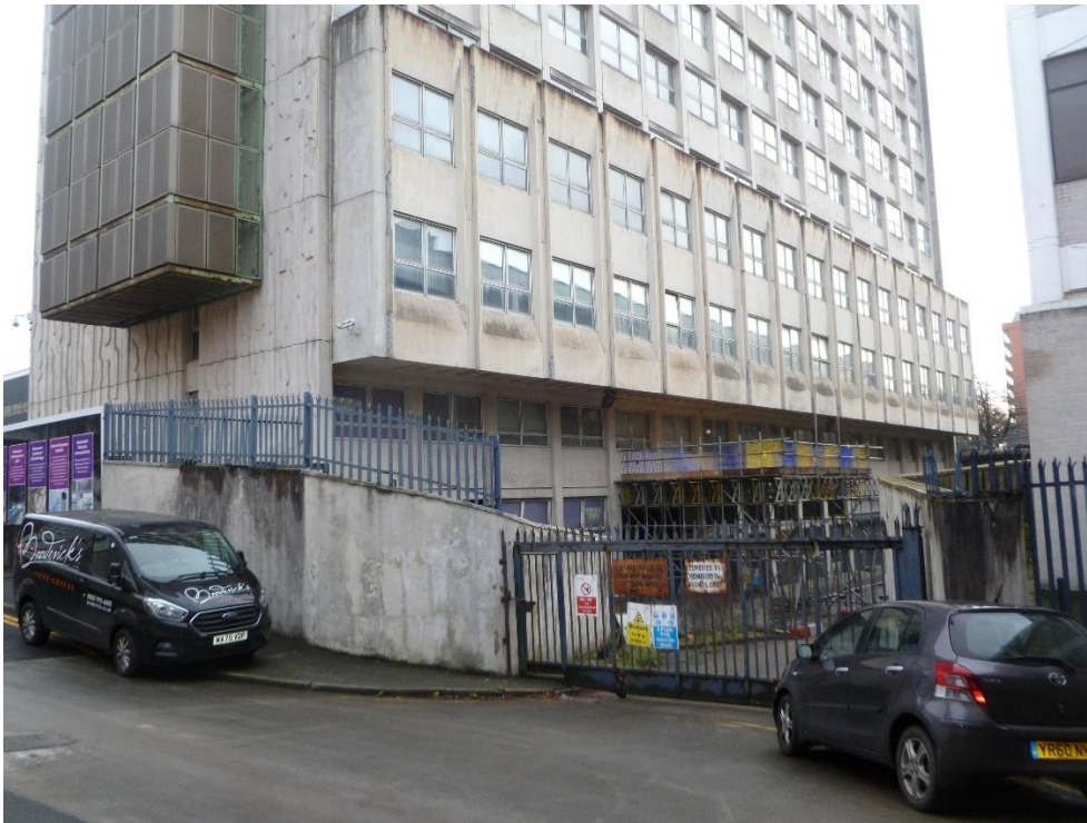
Rear of building, looking south from Drover Lane.
