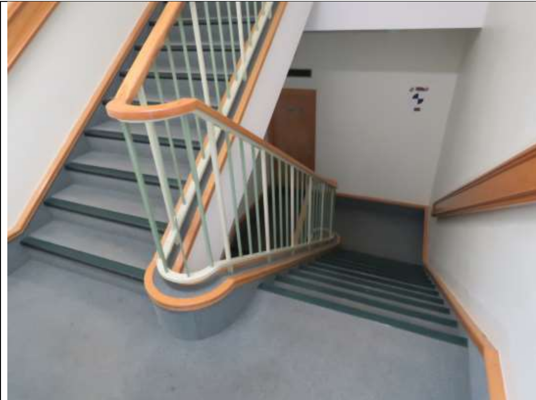
23-32 View in eastern stairwell.
