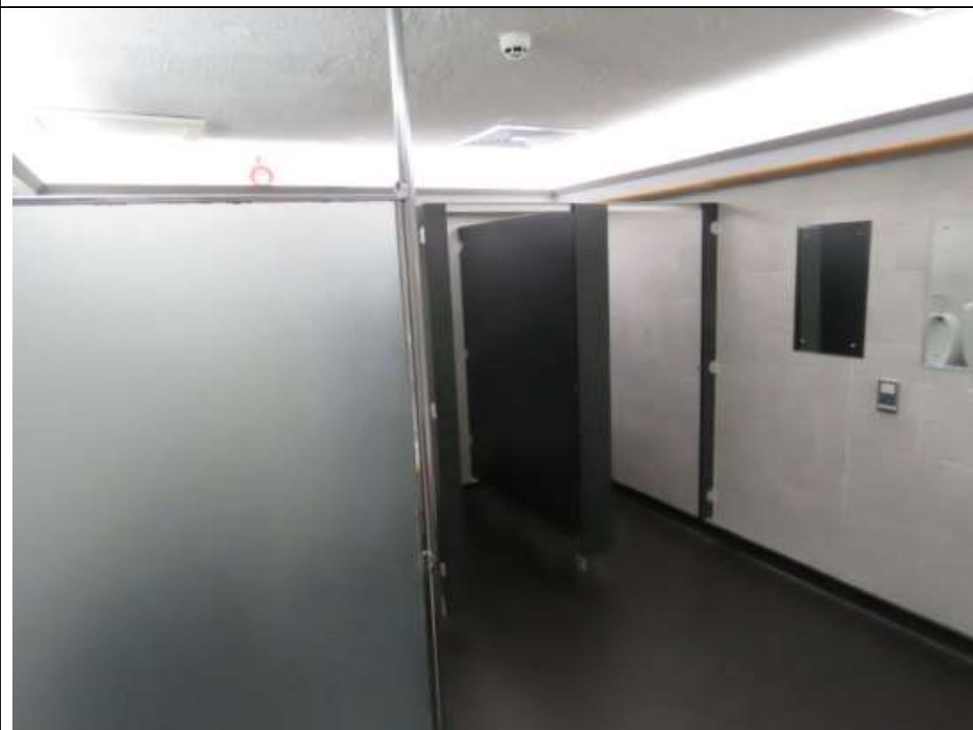
23-35 View in male toilet with original obscured glass screen and non-original cubicles.
