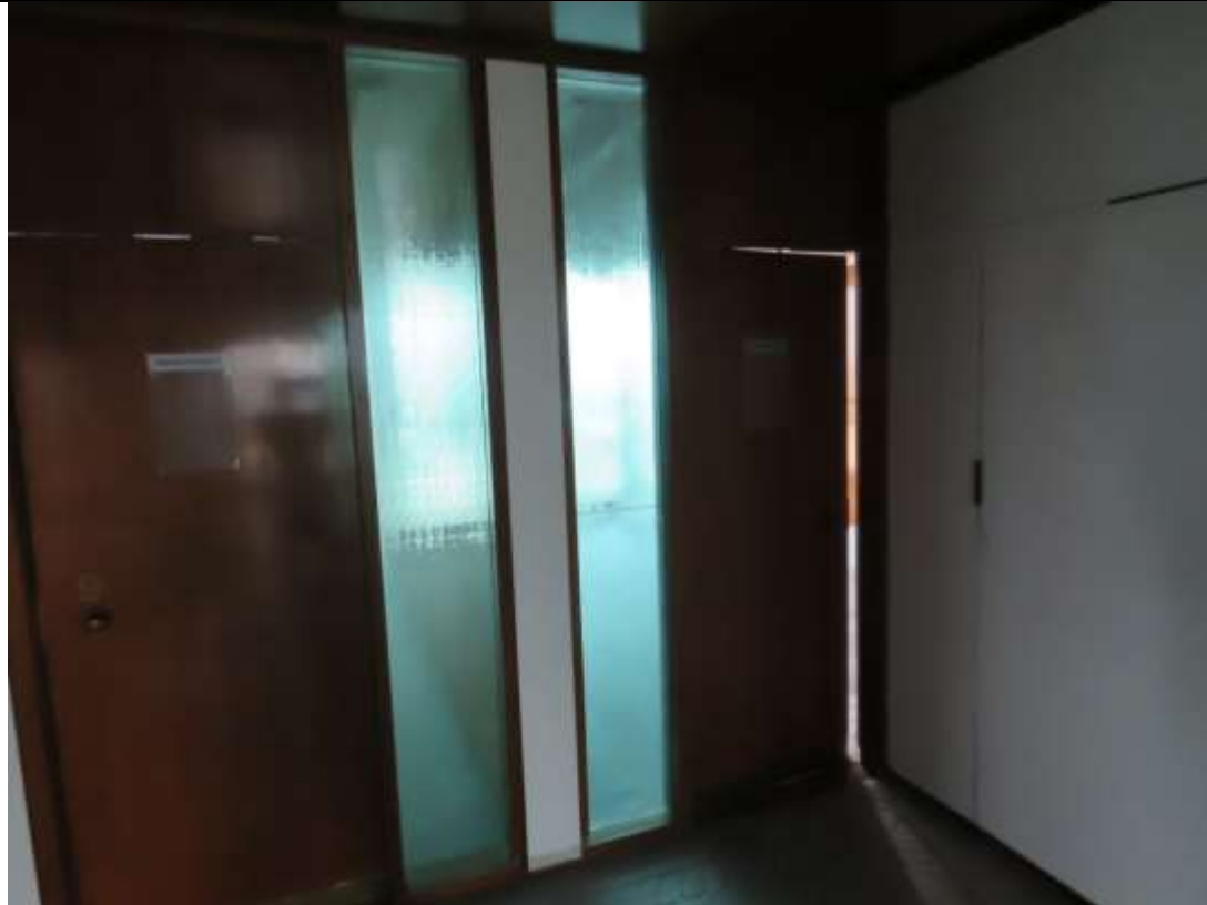
23-18 View of glazed panels and doors to offices 2 and 3.
