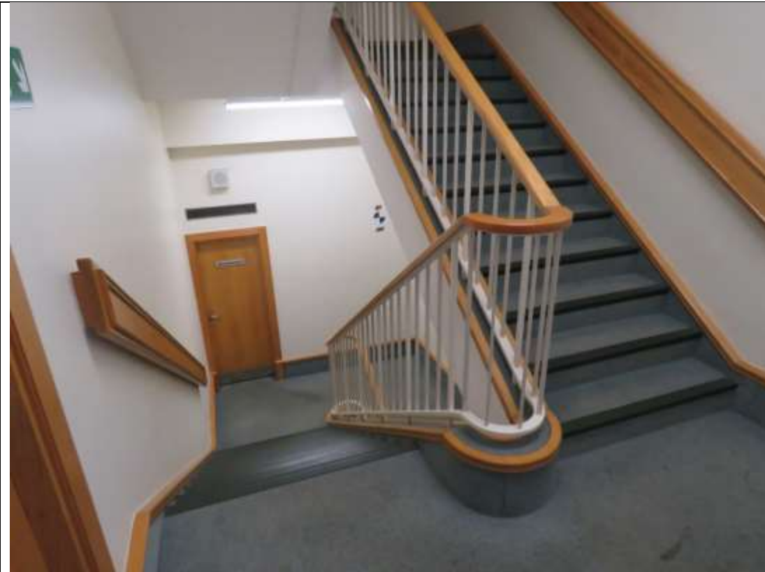
23-34 View in western stairwell.
