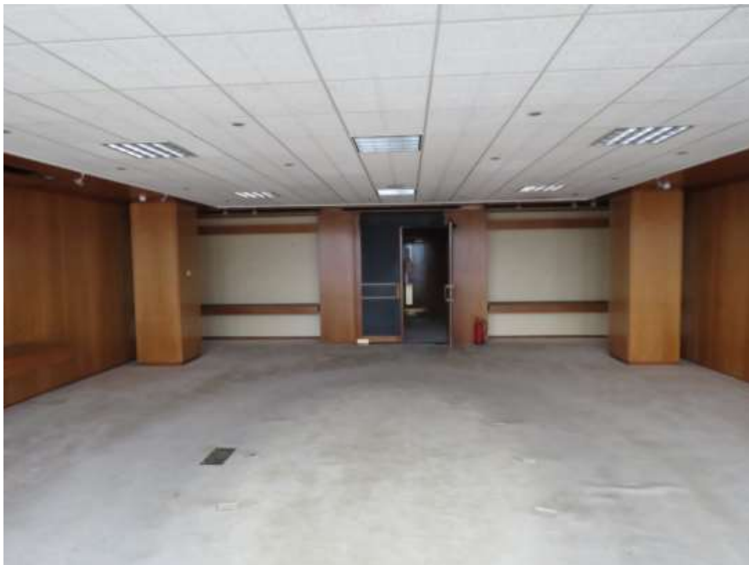
23-07 View south across board room.
