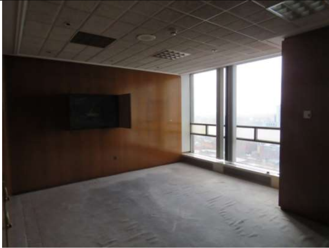
23-22 View east in “Committee Room 1” showing built in chalk boards that are present in every meeting room.
