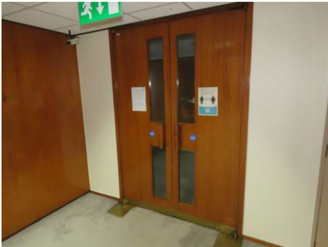
23-03 View of original timber double doors to office space.
