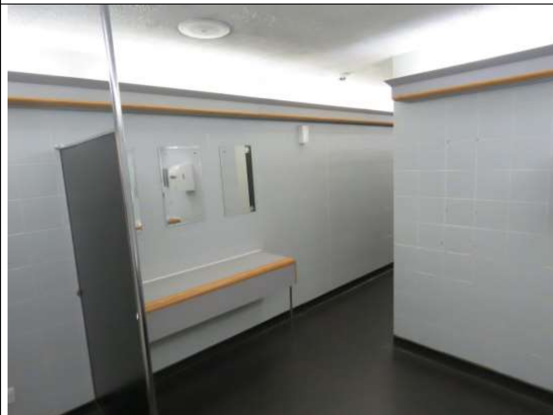
23-33 View in ladies toilet looking towards vanity unit and mirrors.
