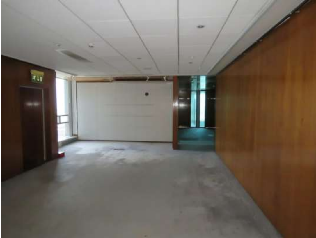
23-08 View within foyer looking west towards the secretary desk, now removed.
