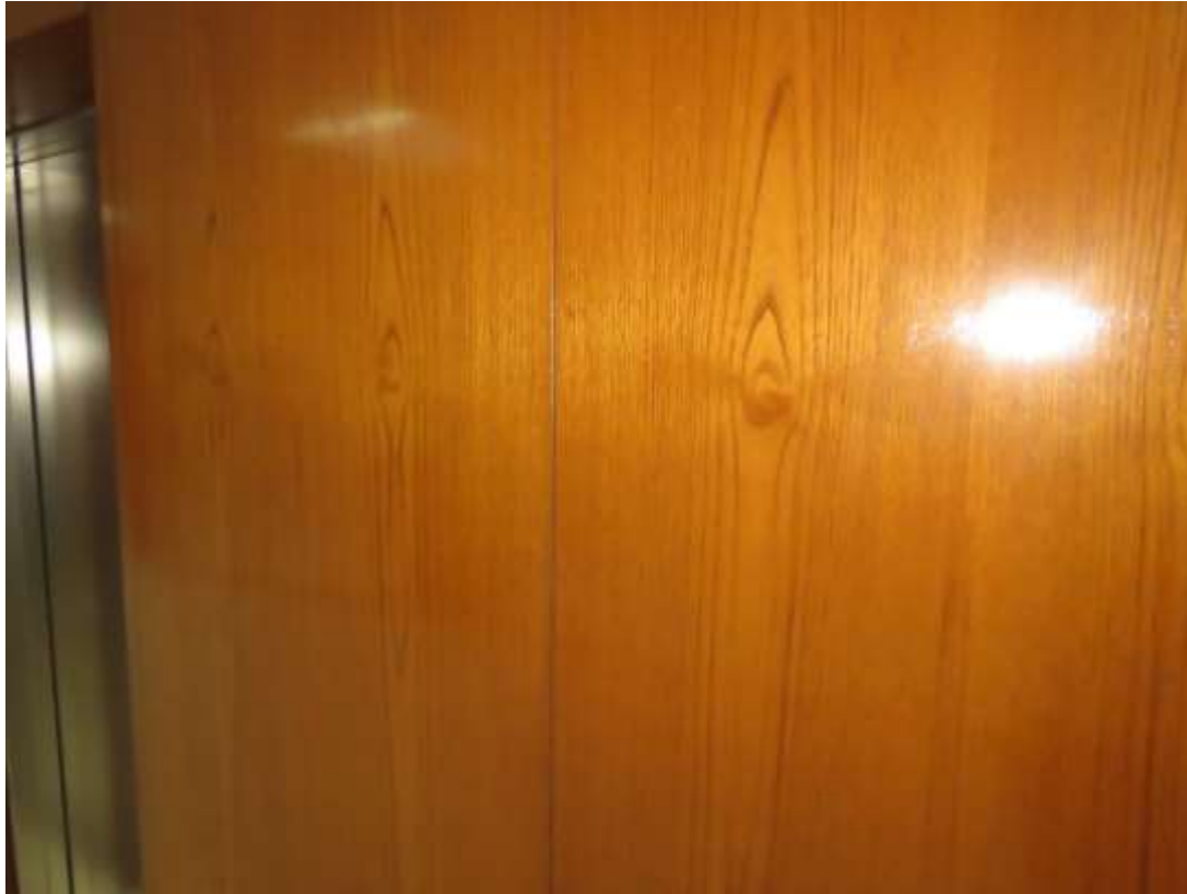
23-02 View of original timber panelling in lift lobby.
