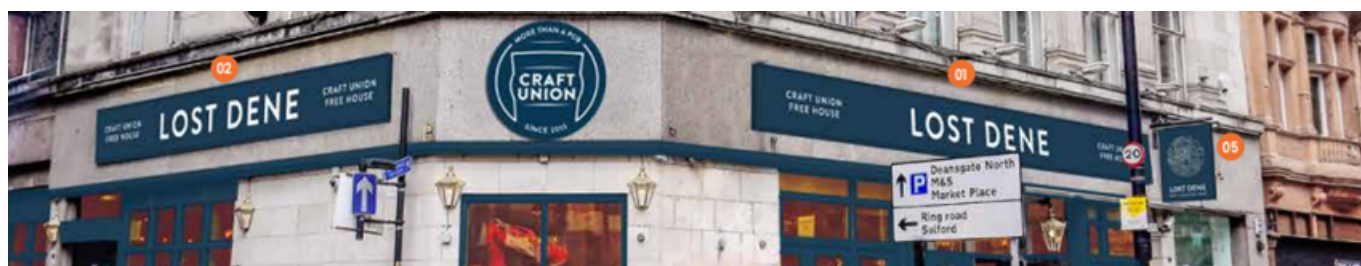
Signage which was installed on the chamfered corner
