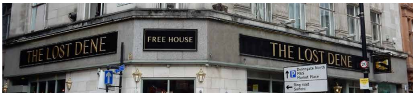
Previously installed signage on the chamfered corner
