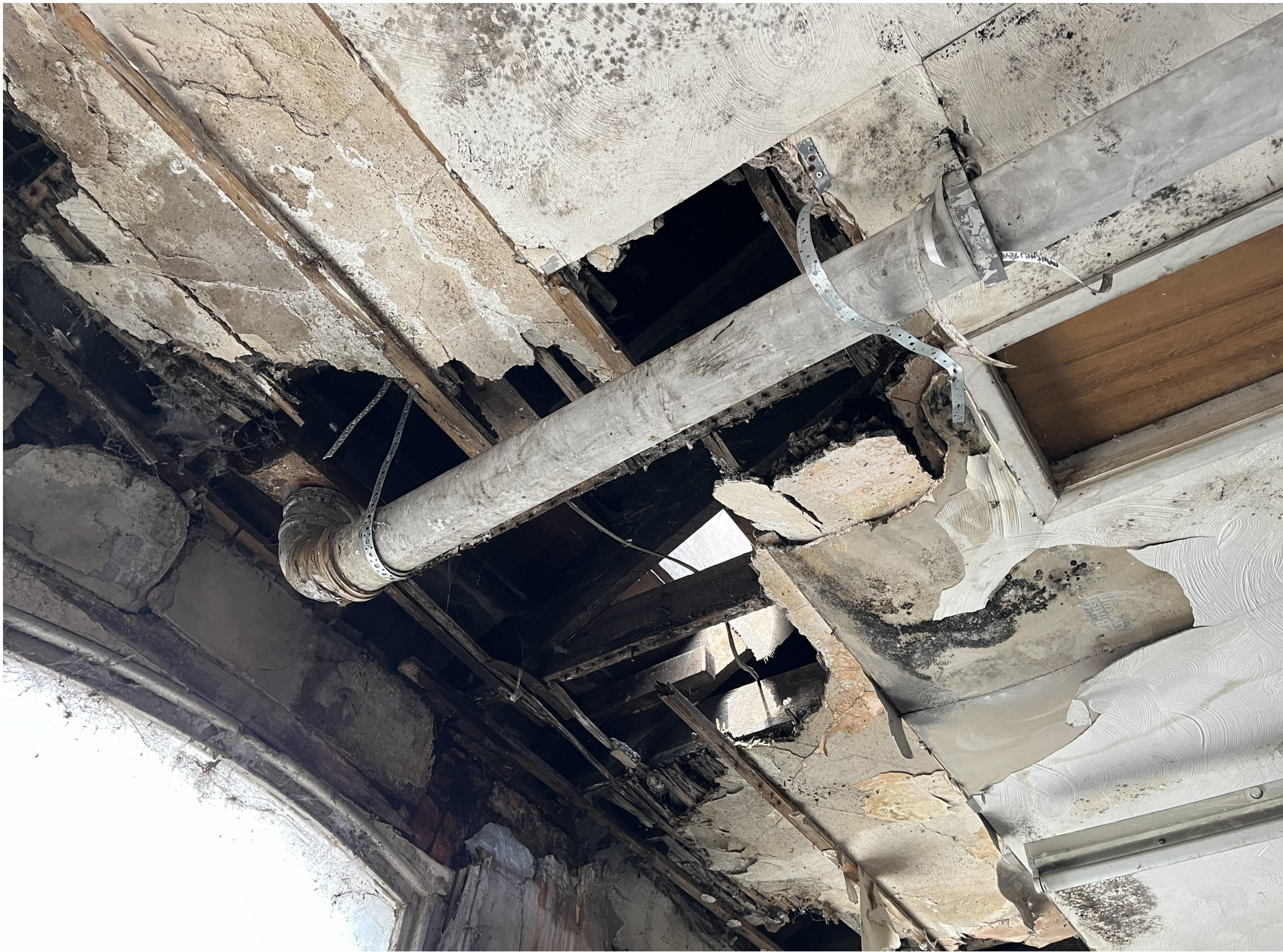
IMG_0443 (Underside of roof - No.68)
