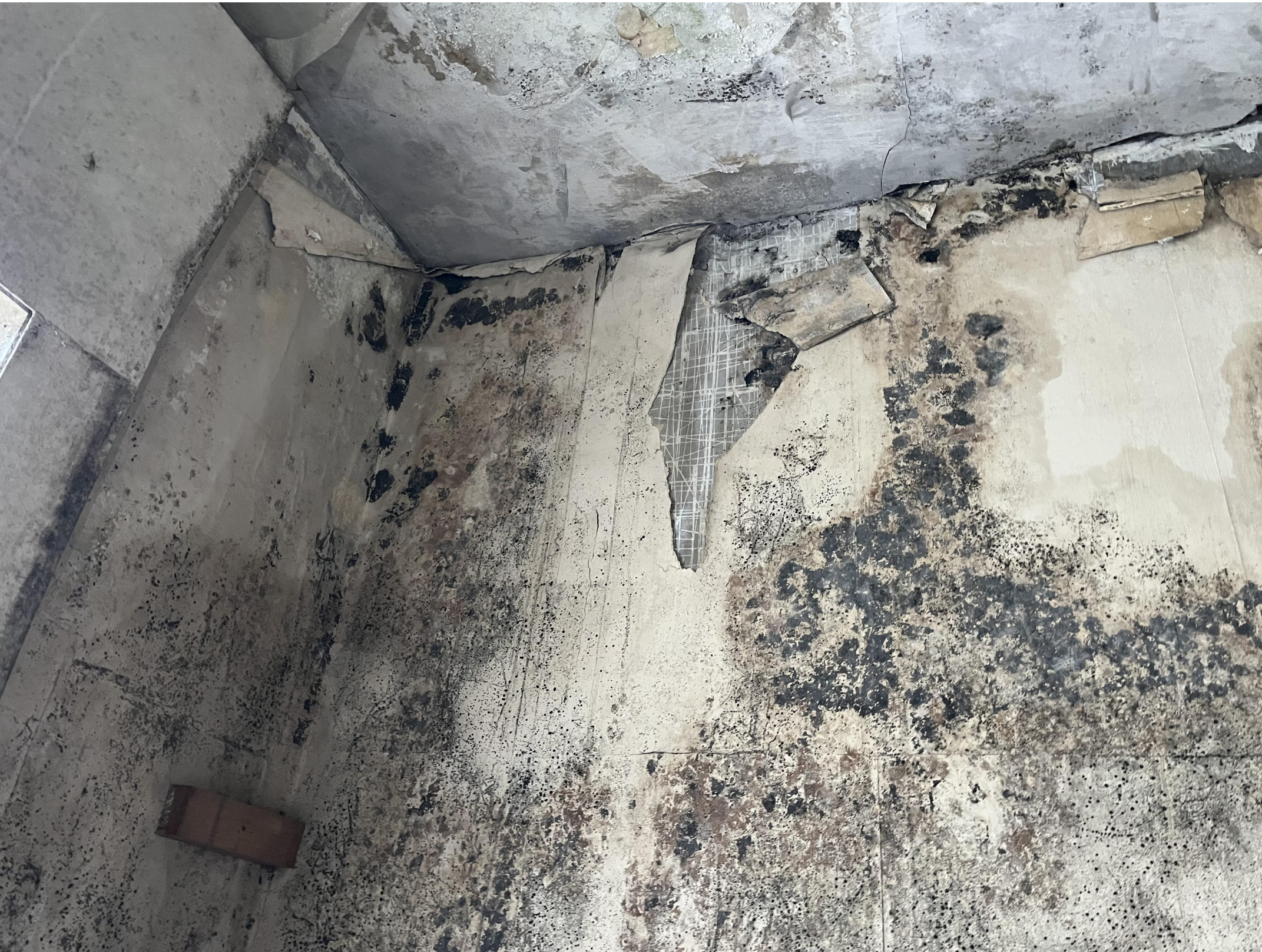
IMG_0414 (First Floor - Internal dividing wall from No.68 side)
