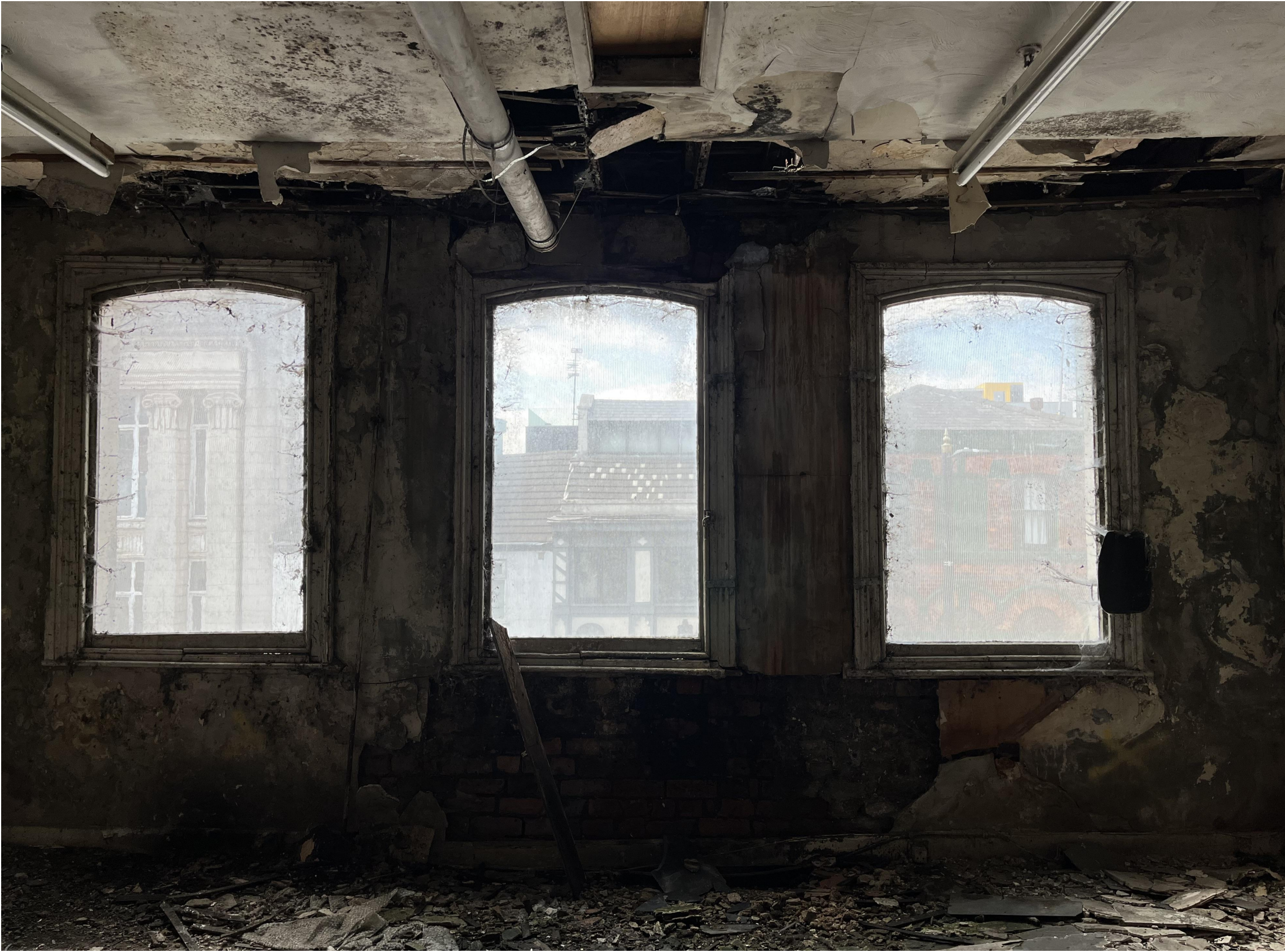
IMG_0440 (Second Floor - No.68 facade)
