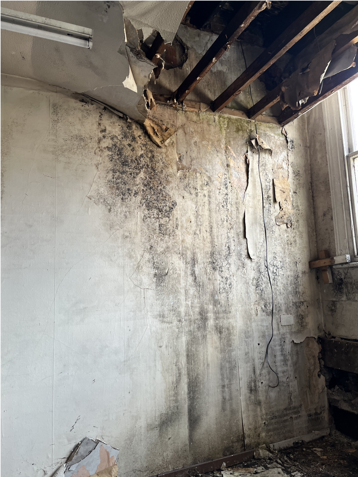
IMG_0414 (First Floor - Internal dividing wall from No.70 side)
