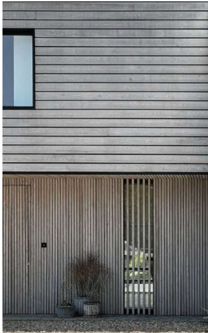
Similar cladding orientation change from horizontal to vertical (Proposed extension will be horizontal to bottom and vertical to top)
