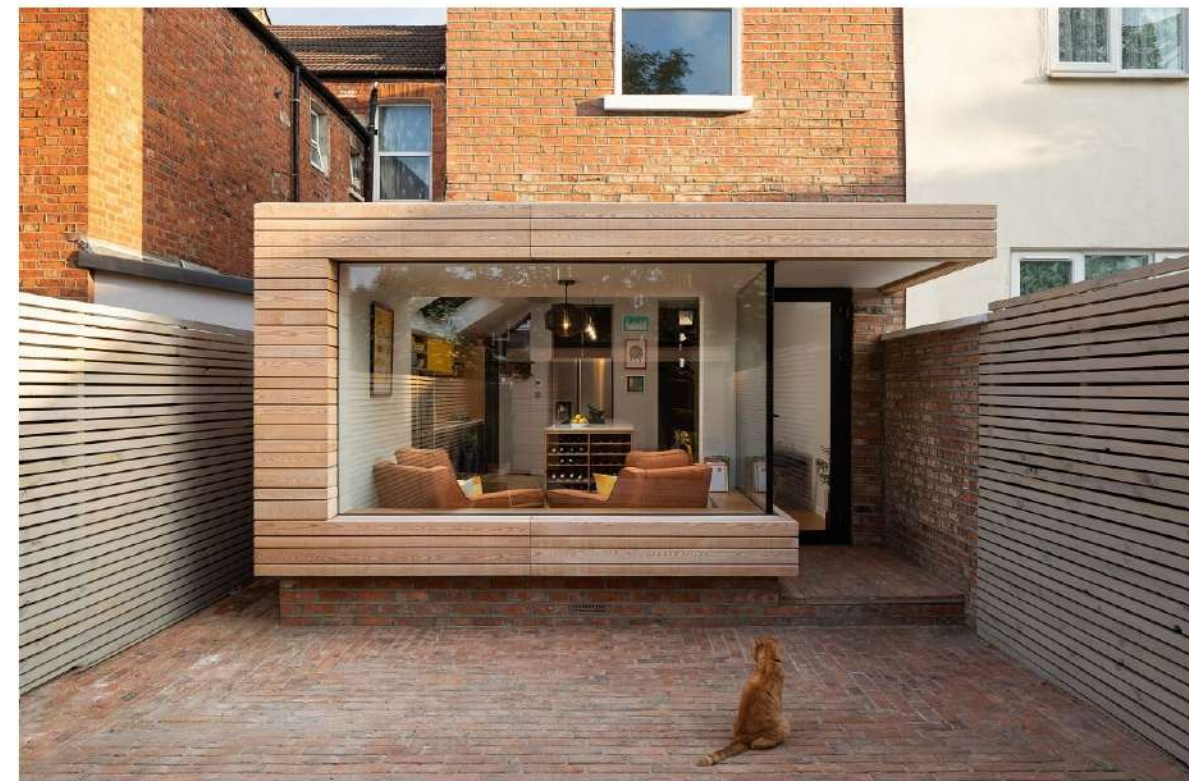
Siberian larch cladding with brick plinth - horizontal orientation and flat roof
