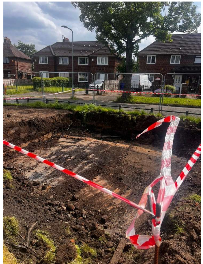
Pictures of location WS101 marked out and excavated to natural clay strata.
