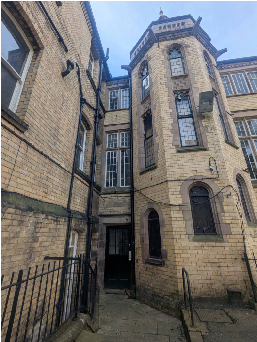
External Escape Door and Location/ Elevations
