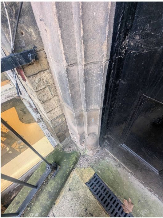
External Escape Door and Stone Surrounding Details
