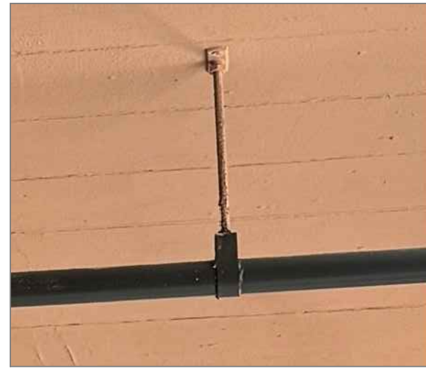
PUMPED WASTE CEILING FIXINGS REFERENCE IMAGE
