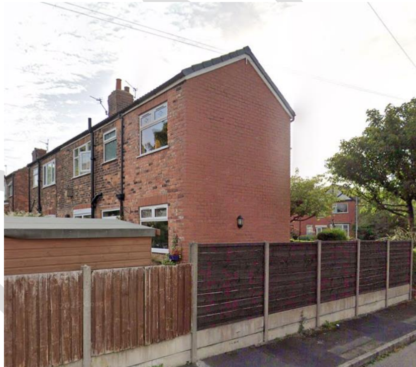
Figure 14 - 41 Grange Park Road
