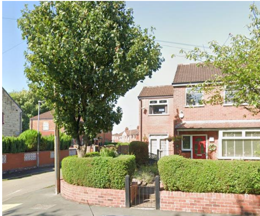
Figure 13 - 41 Grange Park Road
