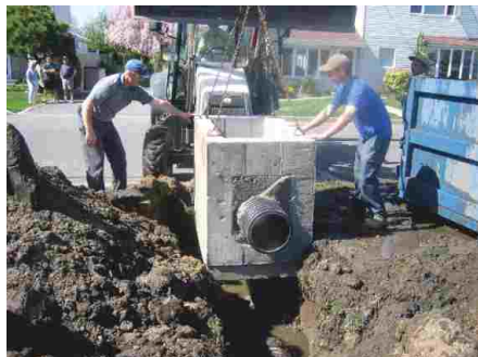
Smaller Smart Filter® being lowered into position
