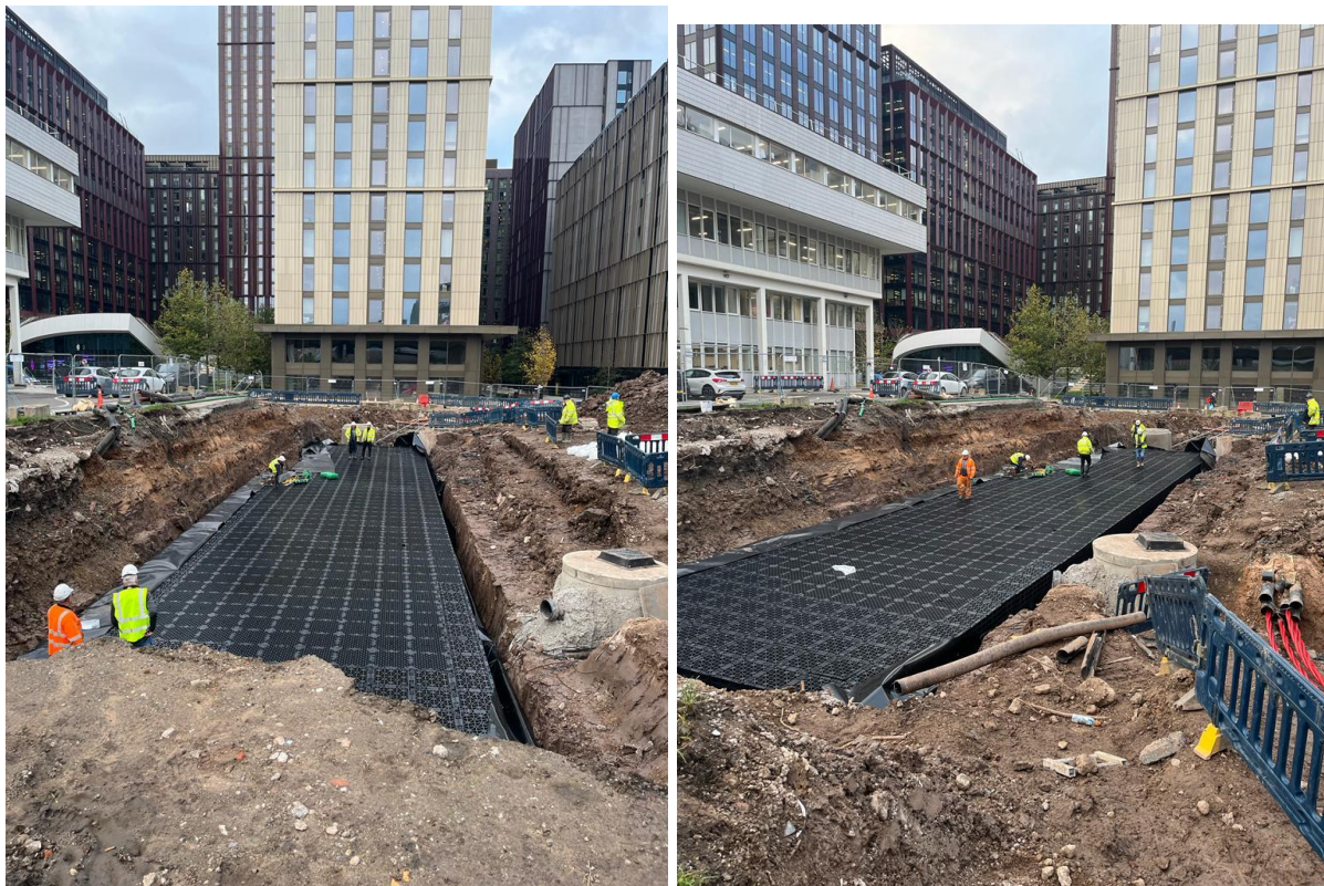
Figure 2 - Attenuation Tank Installation
