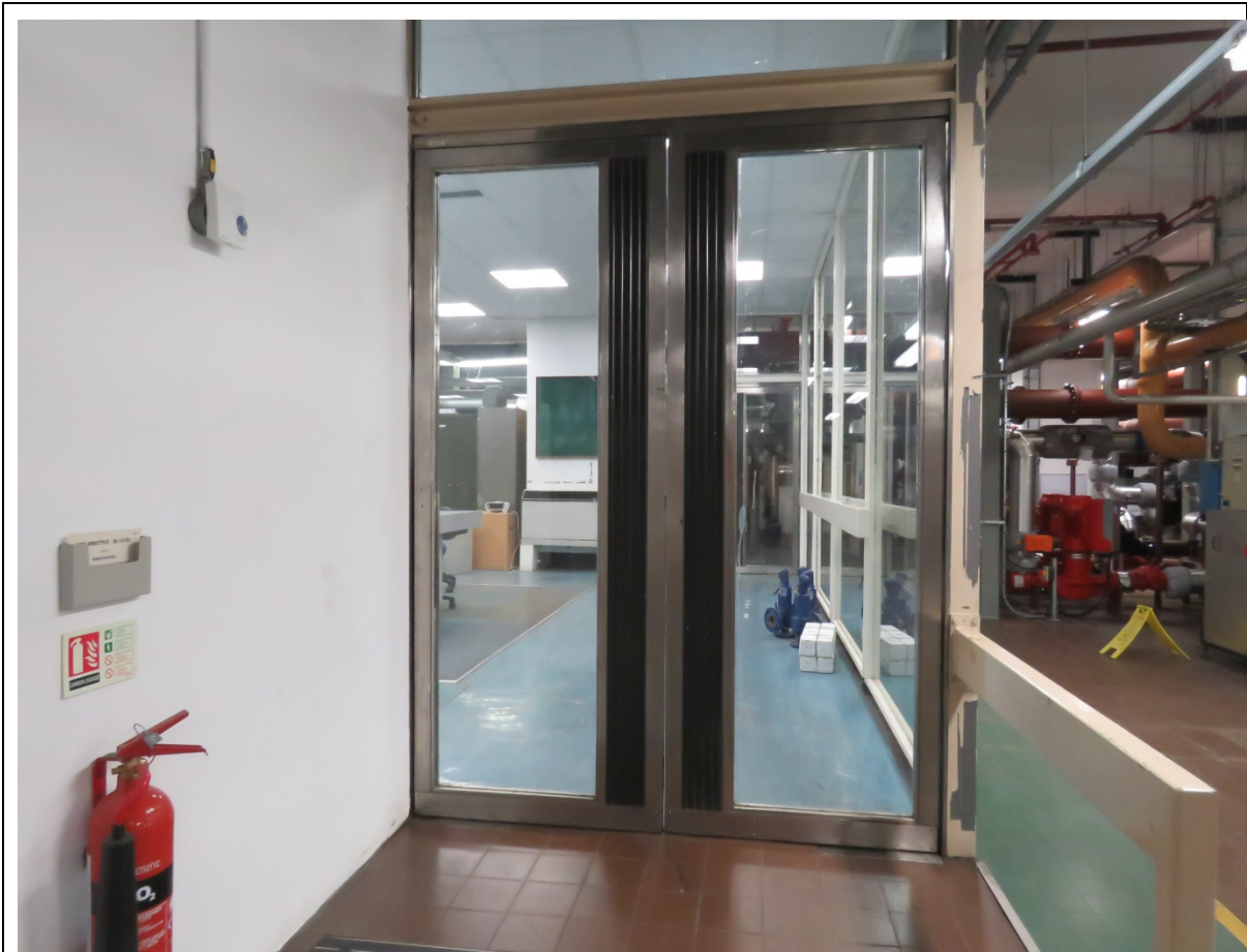
B3-10 View of the original control room doors.
