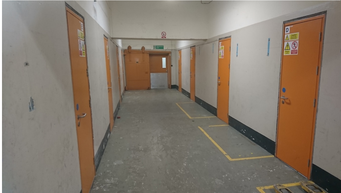
B3-02 View looking east with the doors to each lift pit directly under the each lift above.
