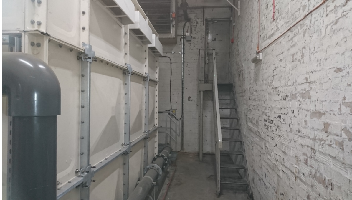
B3-06 View of a steel staircase to one of the external fire exits.
