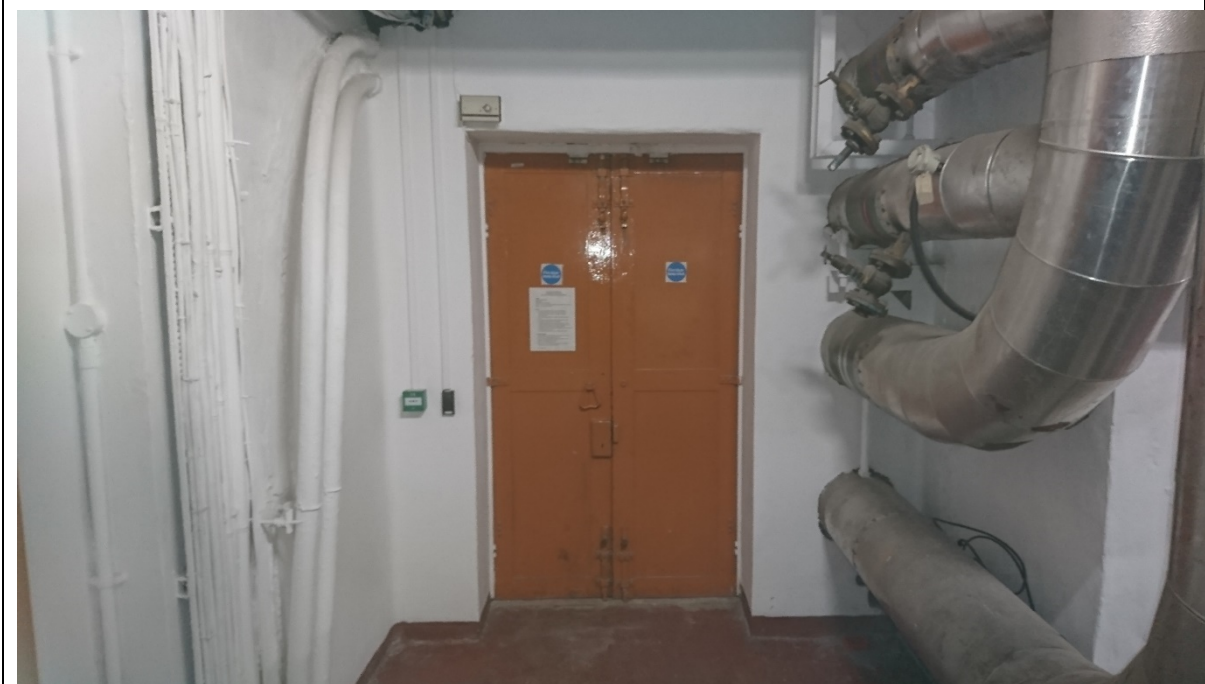
B3-15 View of original steel doors.
