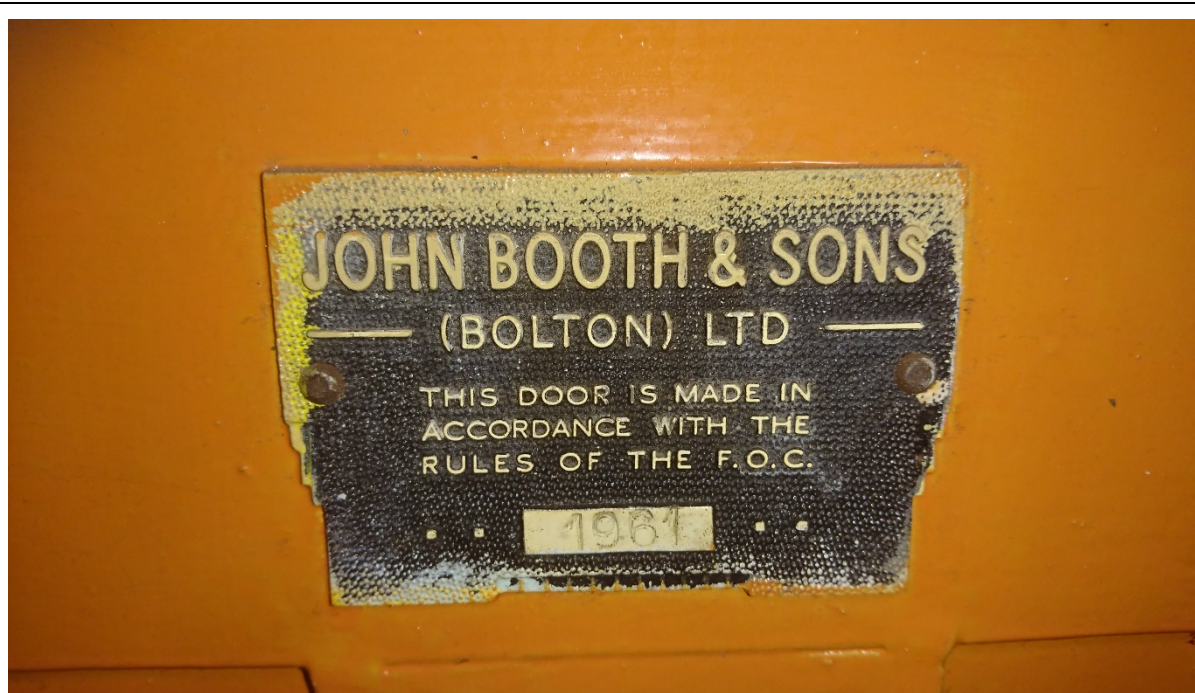
B3-04 Original makers plate on the fire door of John Booth & Sons (Bolton) Ltd.
