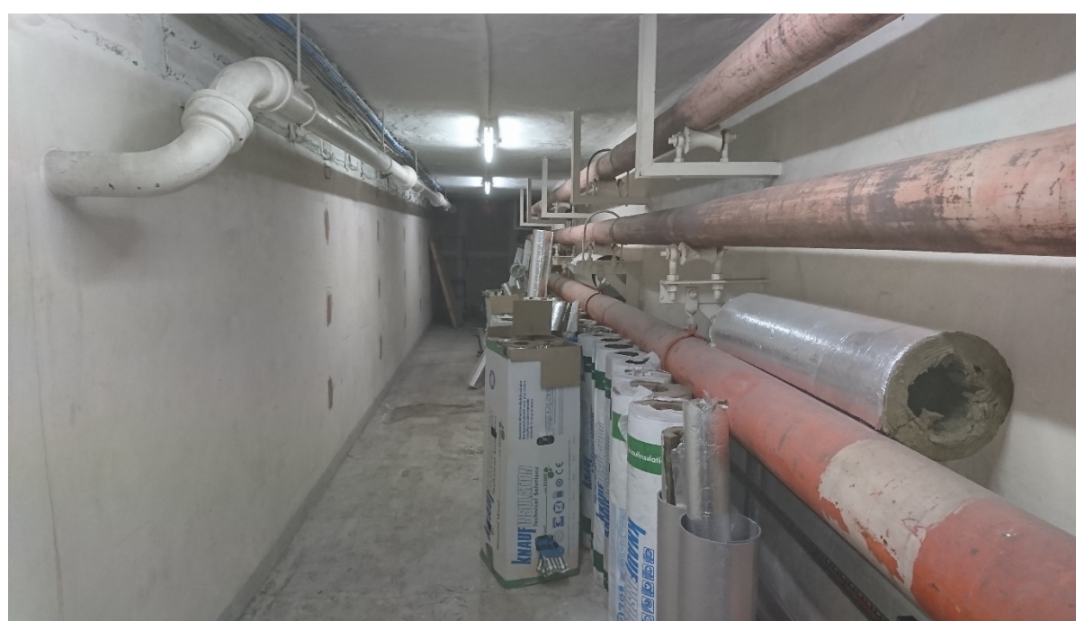
B3-12 View looking north in the underground corridor that connected the CIS tower to New Century Hall and New Century House, now blocked off.
