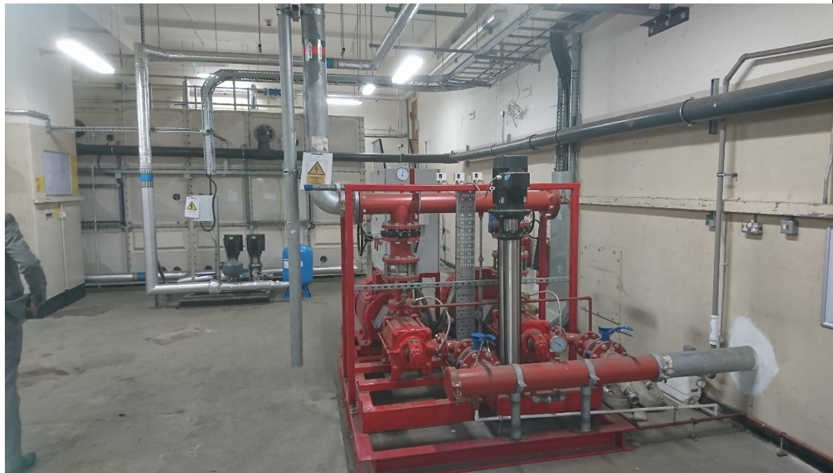
B3-07 View east of the non-riginal plant equipment.
