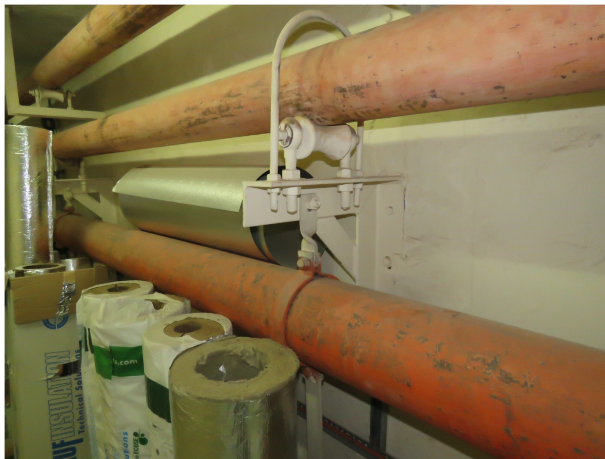
B3-13 Detail of the roller support to pipework that connected the plant of the CIS tower to New Century House.
