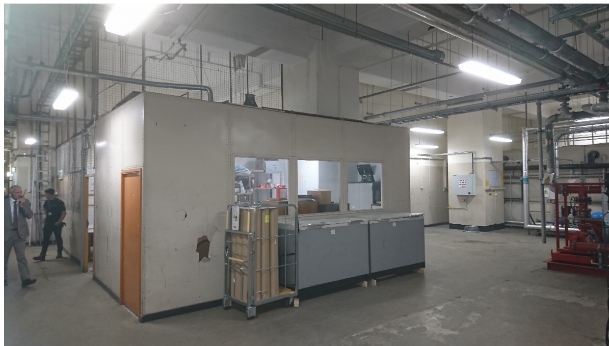
B3-05 View looking north east of one of the non-original offices that have been inserted into the basement.
