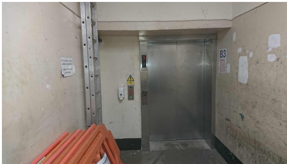
B3-01 Looking north-east towards the service lift.
