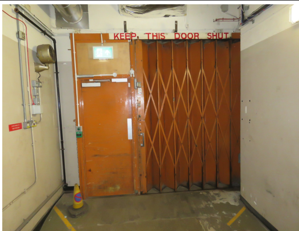
B3-20 View south looking at the lift door and shutter.
