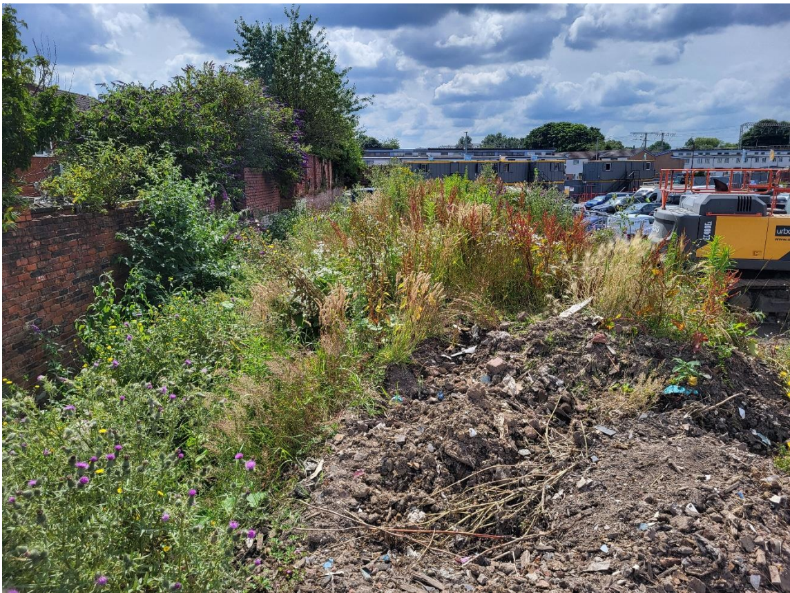
Pic 6 – Spoil stockpiles along eastern boundary
