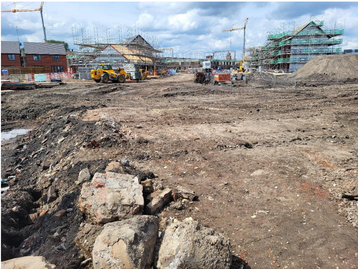
Pic 2 – Construction works currently underway to western portion of site
