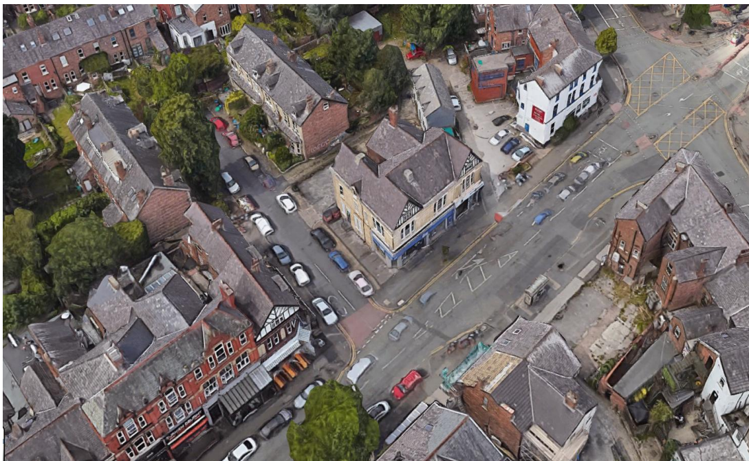
Image 5: Overhead view of site facing north west.
