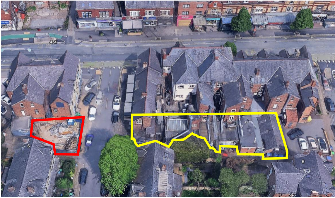
Image 6: Overhead view showing the proposed development site (red) and large commercial rear extensions in the immediate vicinity (yellow)
