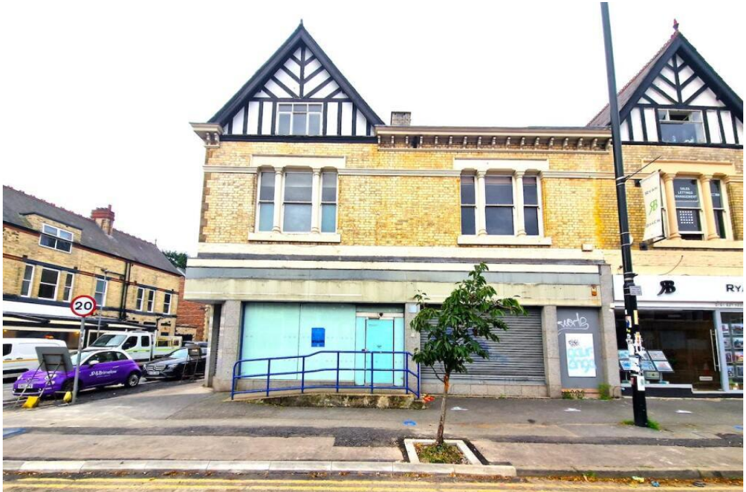
Image 2: Photograph of front elevation from Barlow Moor Road prior to the approval of Ref 140033/FO/2024.
