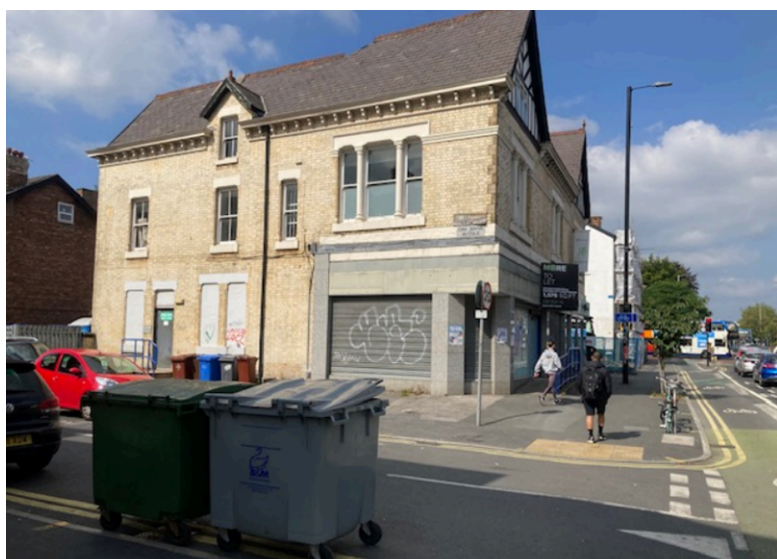
View of application property form Barlow Moor Road
