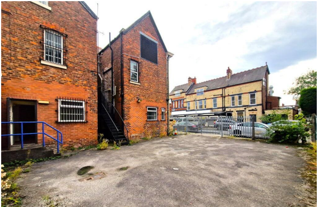
Image 3: Photograph of rear elevation and car park facing towards Silverwood Avenue.
