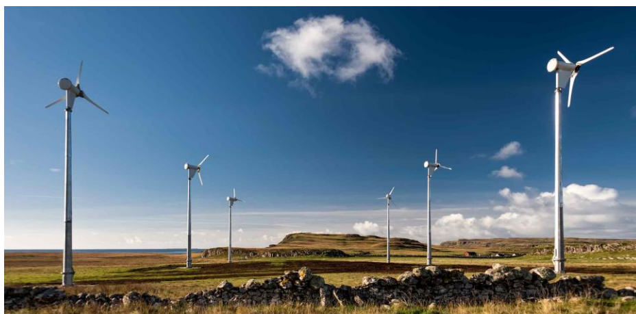
Figure 13: Typical Small Scale 6kW Wind Turbine
