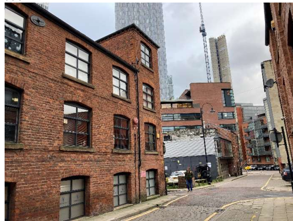
Fig A2.4: View of site from Little Peter Street looking west.
