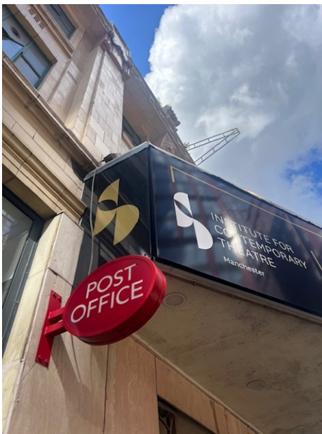
Figure 4 – Existing fascia panel
