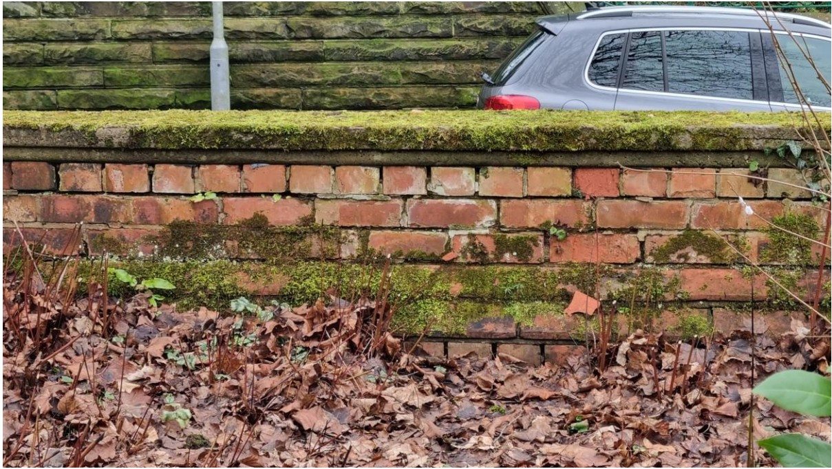
Photo 8: Photograph shows the parapet wall section on the Parsonage Garden side.
