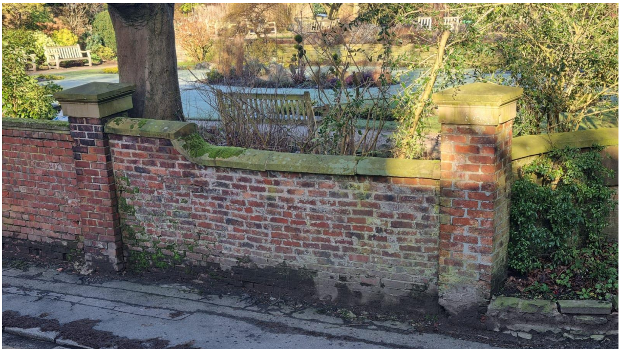
Photo No.9: Photograph shows the section of wall between the two piers with original coping stones.
