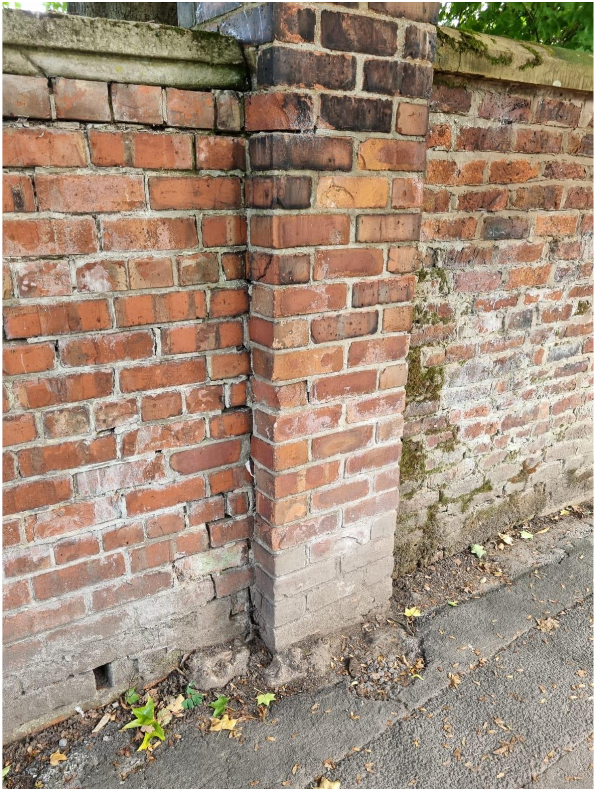
Photo 3: Photograph shows pier adjacent Field Maple tree and the two different brick bonds either side, English Garden Wall bond and Stretcher bond.
