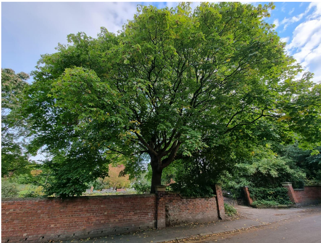
Photo 1: Photograph taken on Stenner Lane facing the Western perimeter boundary retaining wall to Fletcher Moss Art Gallery. Photo shows section of wall to be dismantled and rebuilt adjacent the large Field Maple Tree.
