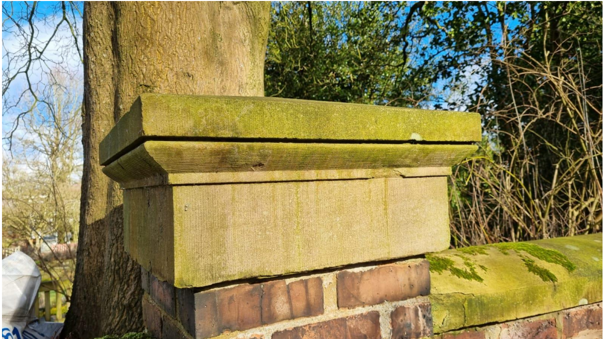
Photo No.10: Photograph shows the existing pier coping.
