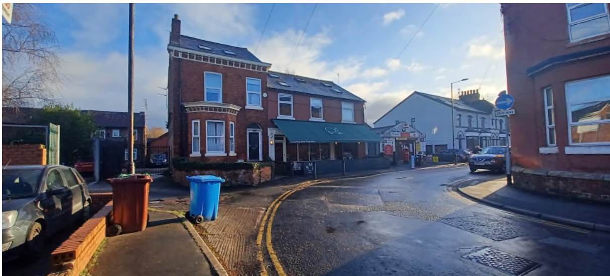
Application property in December 2024
