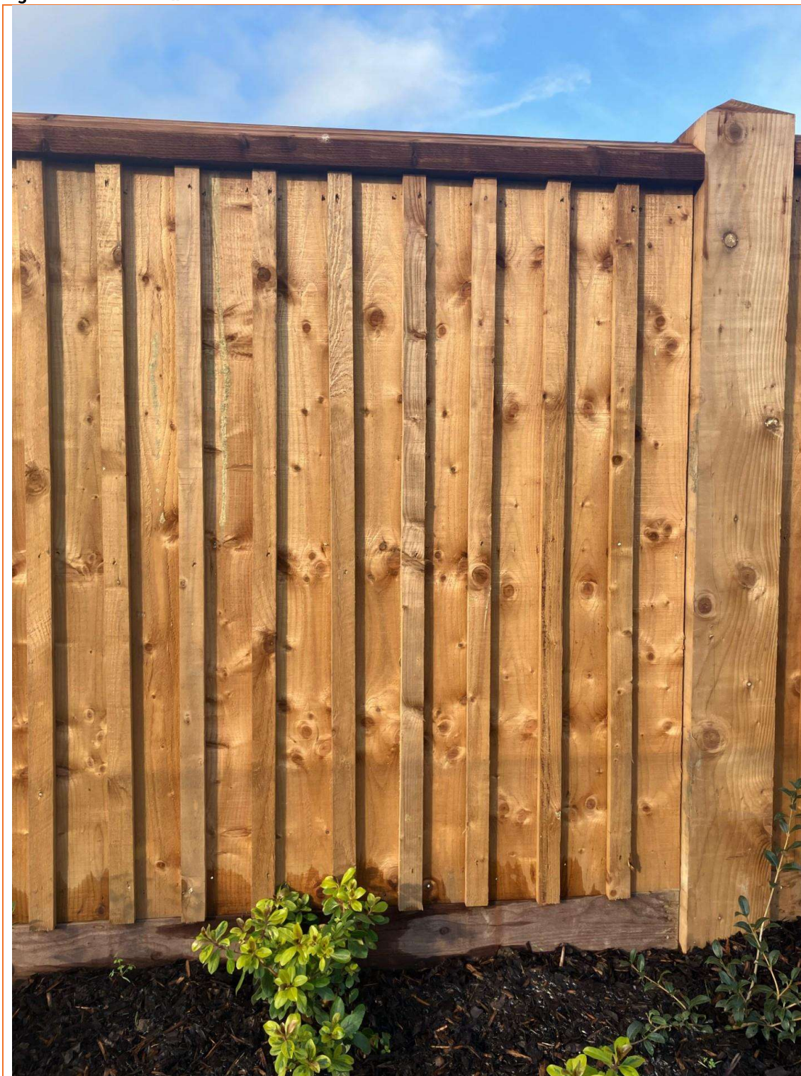
Figure 2 Installed barrier at Plot 9
