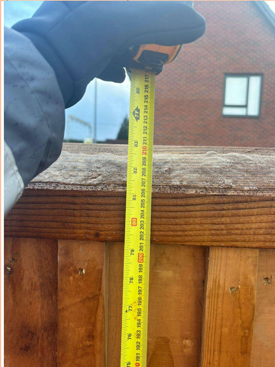
Figure 3 Installed barrier at Plot 9 - height
