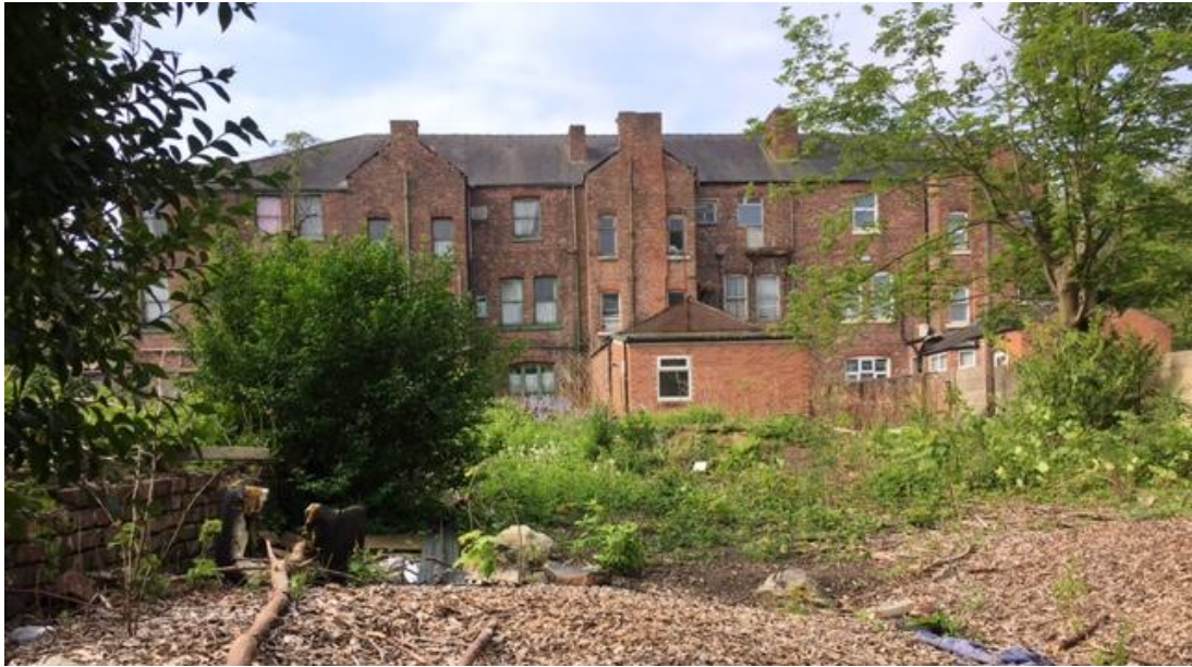
Image 3 – Photograph of rear elevation of site demonstrating imposing scale of the terrace of which the site forms part of
