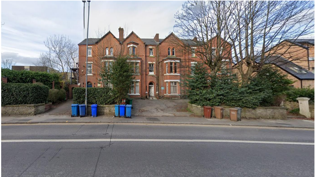
Image 2 – Streetview of site during its previous occupation as a hotel in 2021
