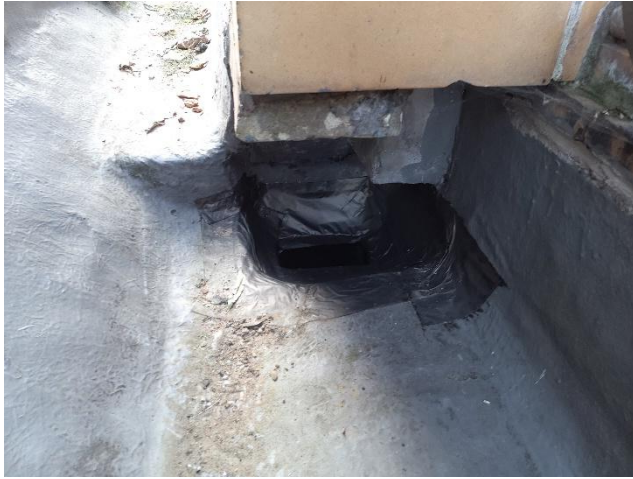
13 Historic repairs, front box gutter
