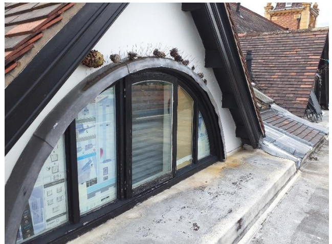
4. Arched windows to rear flat roof
