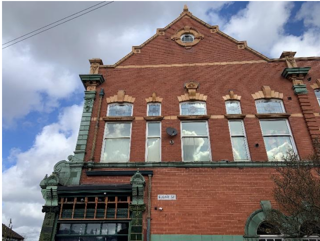
1 View of existing upper windows - Elgar Street
