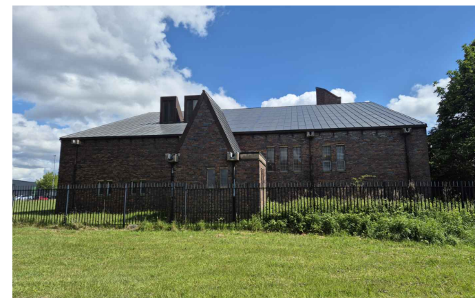
Relevant Area View from South-West
