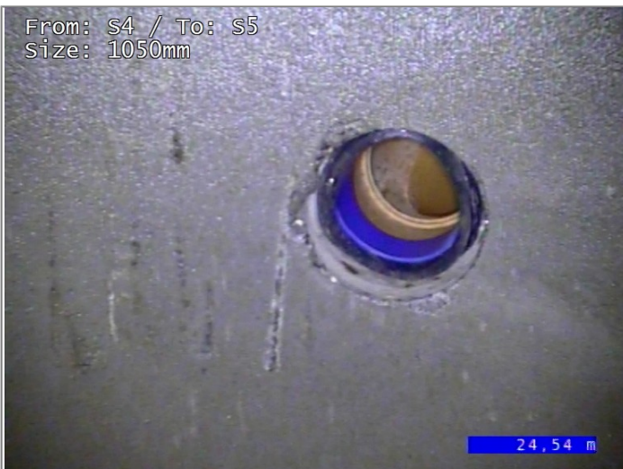
Junction at 1 o'clock, diameter 150mm
