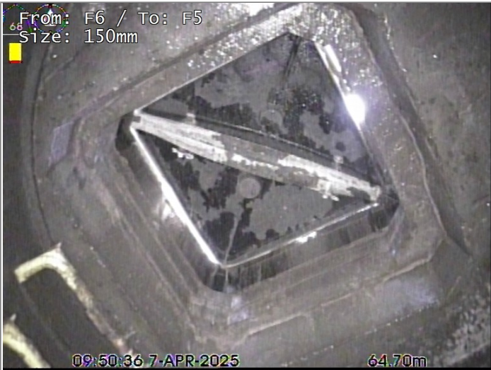
Finish node type, manhole, reference F5
