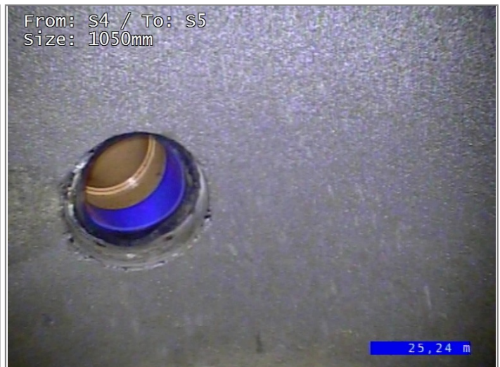
Junction at 11 o'clock, diameter 150mm
