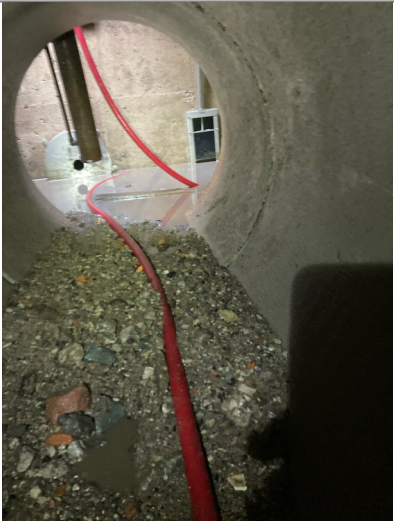
Other Site Photos: General photo
