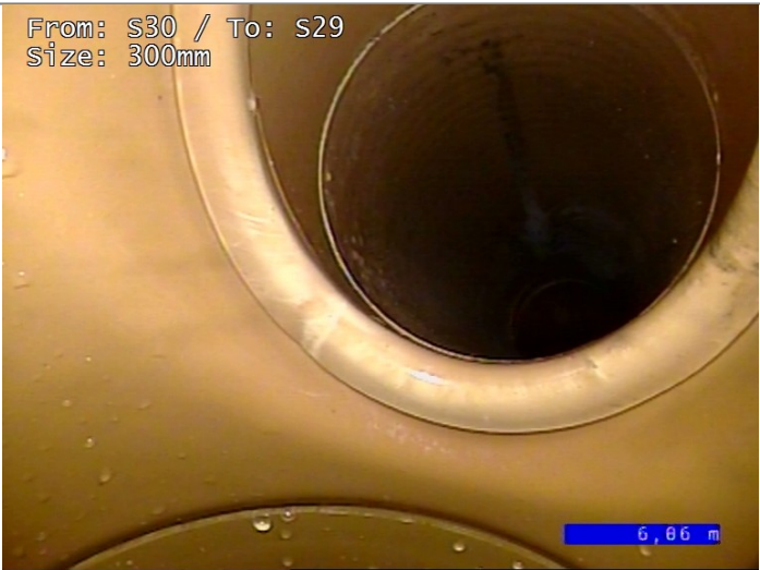
Junction at 1 o'clock, diameter 150mm
