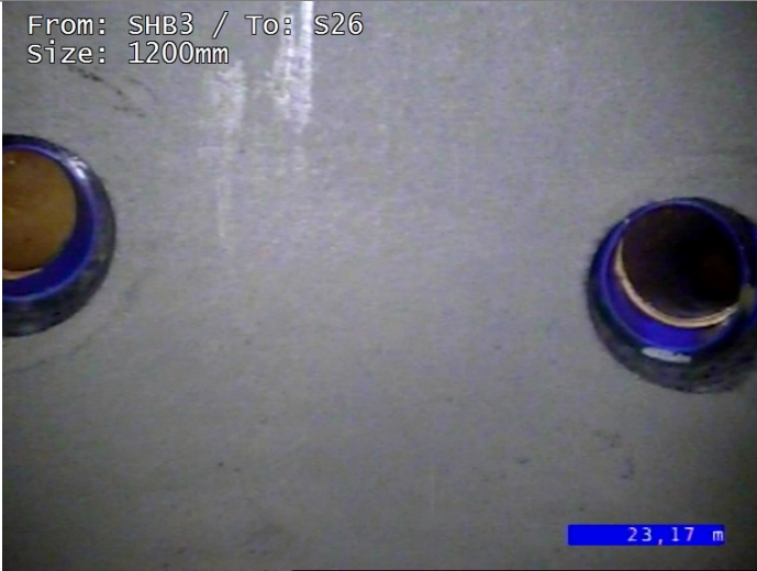
Junction at 1 o'clock, diameter 150mm
