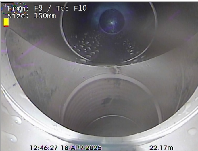
Junction at 6 o'clock, diameter 150mm
