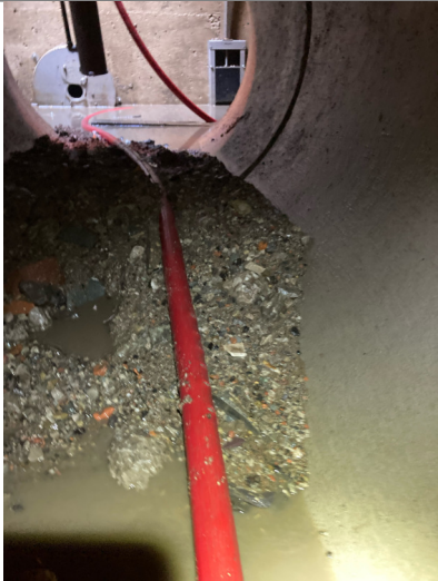
Access problems: General photo
