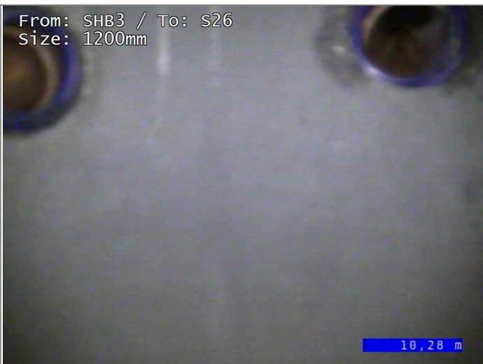
Junction at 1 o'clock, diameter 150mm
