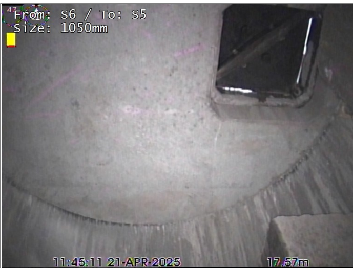
LARGE OFF CUTTS REMOVED BY HAND
