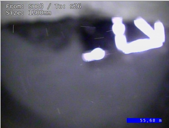
Finish node type, manhole, reference S26
