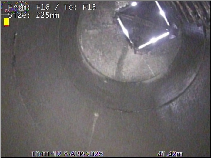
Finish node type, manhole, reference F15
