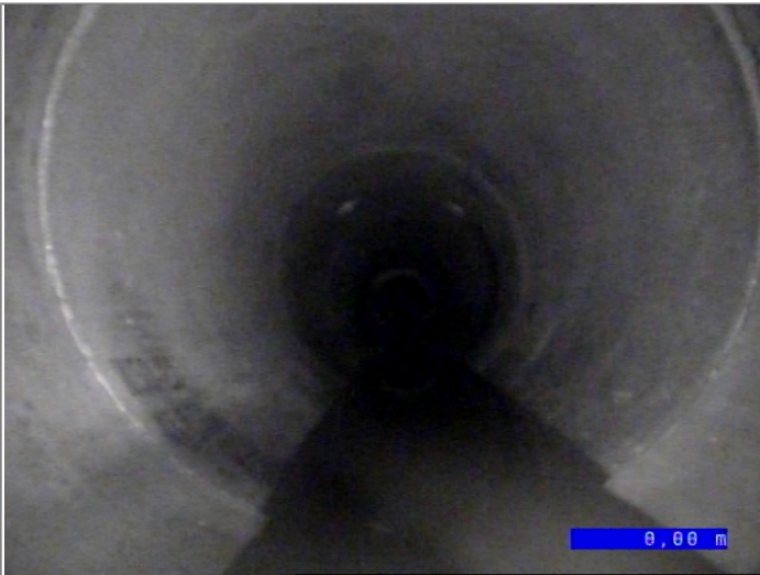
Start node type, manhole, reference SHB2
