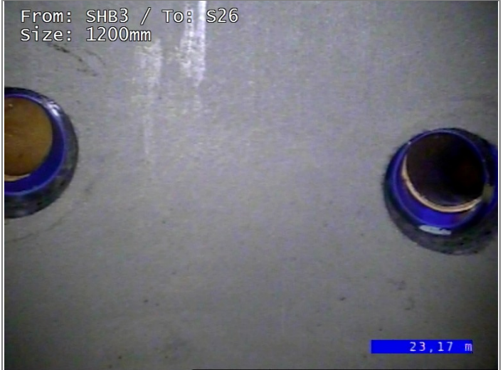
Junction at 11 o'clock, diameter 150mm
