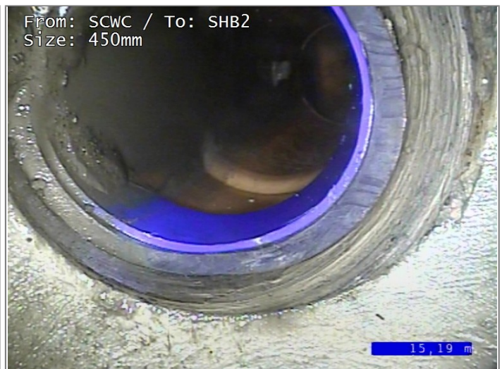
Junction at 8 o'clock, diameter 225mm
