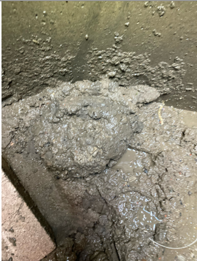
Other Site Photos: General photo
