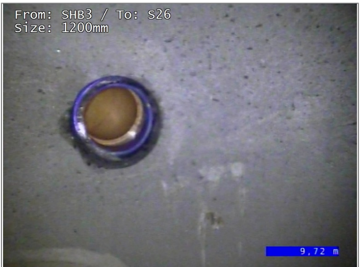
Junction at 11 o'clock, diameter 150mm
