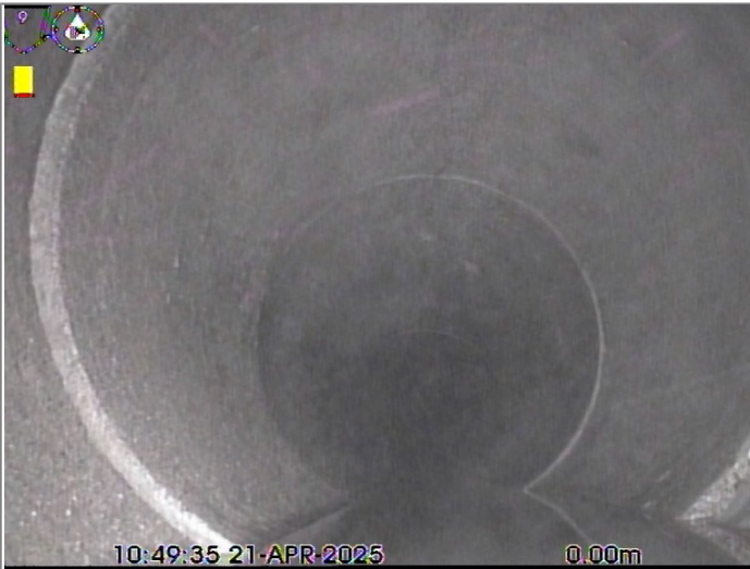
Start node type, manhole, reference S9
