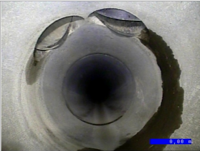
Start node type, manhole, reference S43
