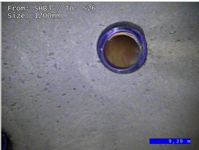
Junction at 1 o'clock, diameter 150mm
