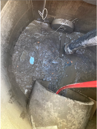
Other Site Photos: General photo
