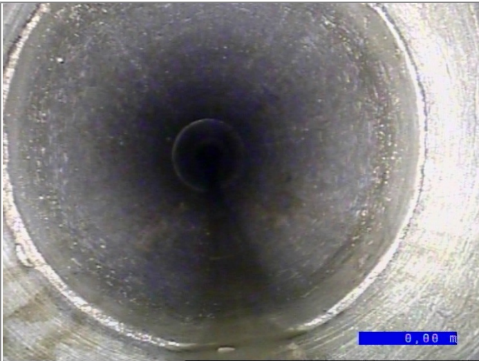
Start node type, manhole, reference S42
