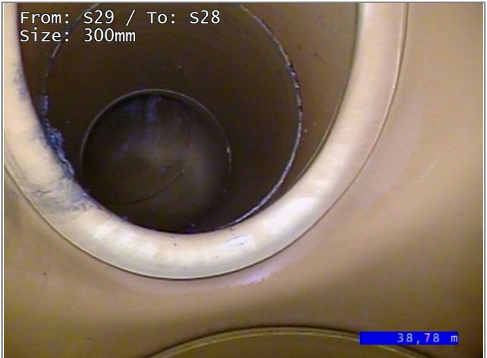
Junction at 11 o'clock, diameter 150mm
