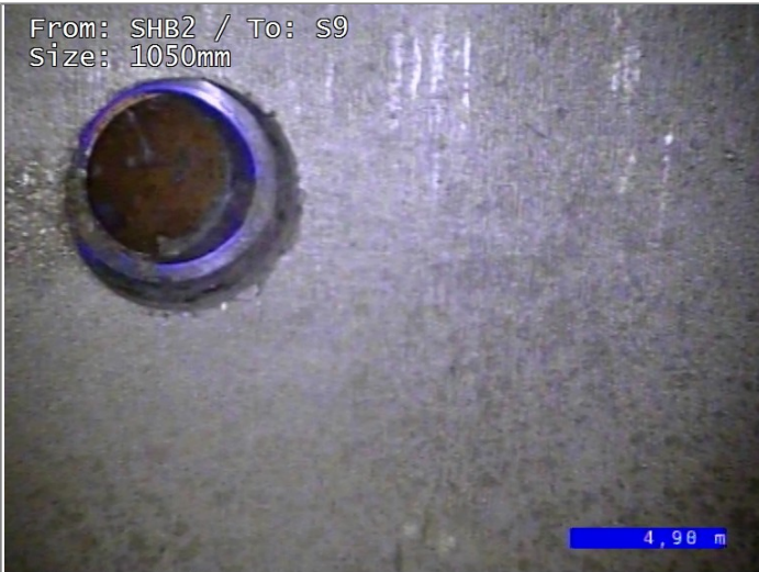
Junction at 11 o'clock, diameter 150mm
