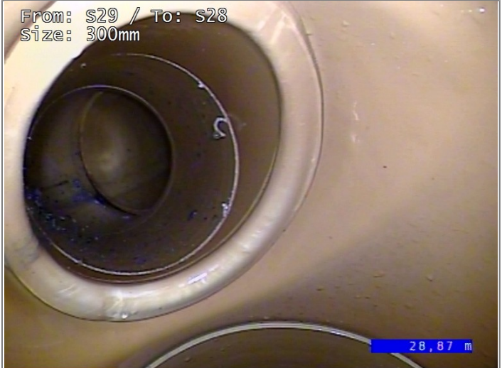
Junction at 10 o'clock, diameter 150mm
