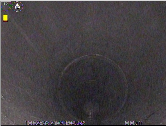
Start node type, manhole, reference S52
