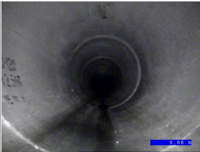
Start node type, manhole, reference S4
