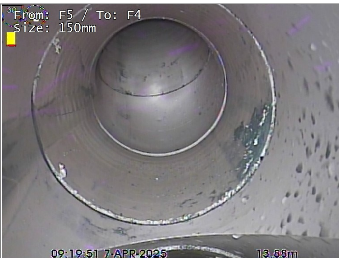
Junction at 9 o'clock, diameter 150mm
