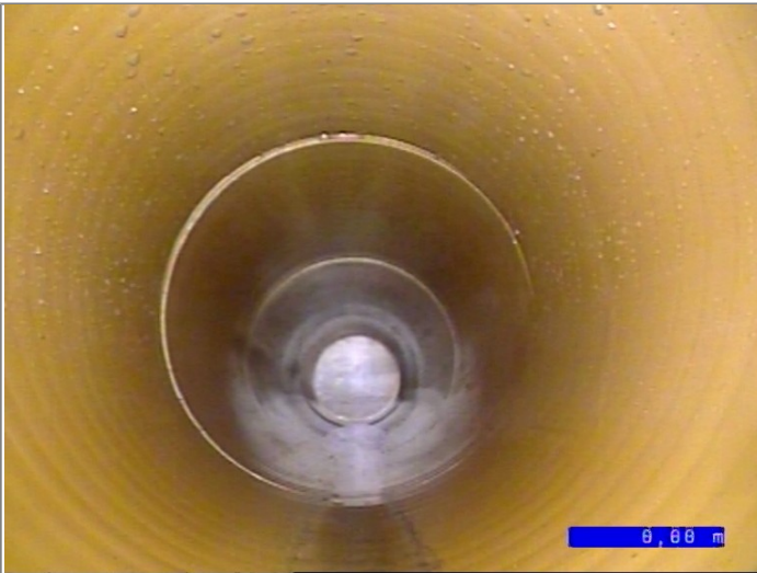
Start node type, manhole, reference S30
