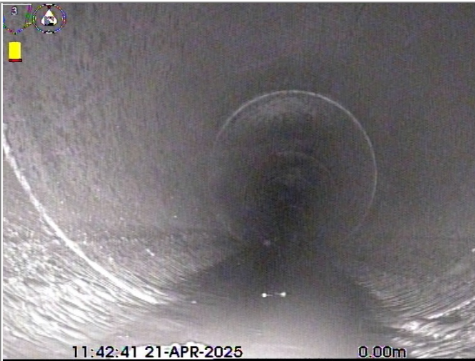
Start node type, manhole, reference S6
