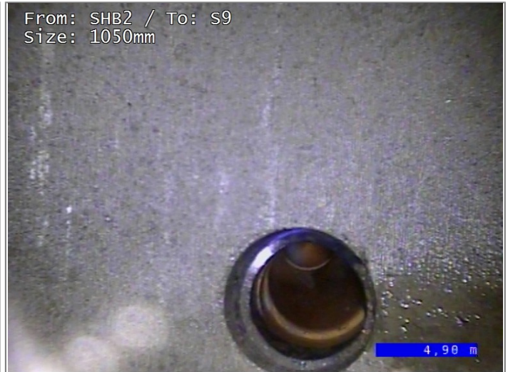
Junction at 1 o'clock, diameter 150mm
