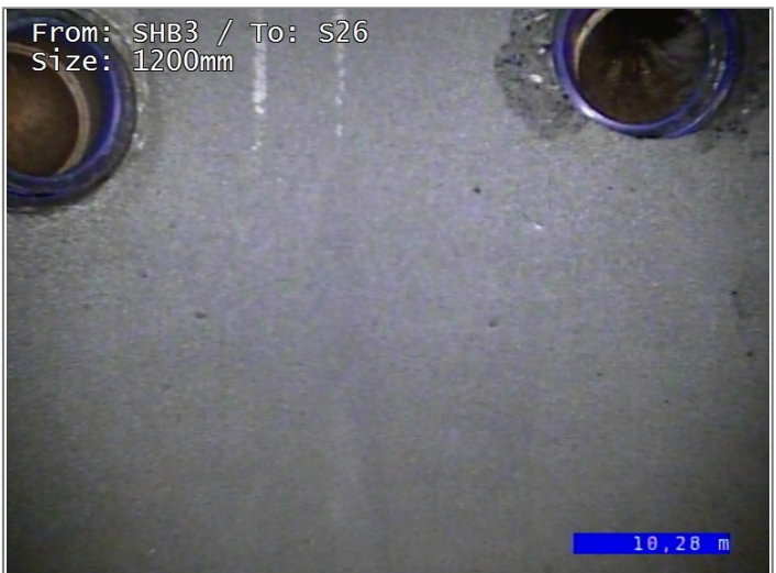
Junction at 11 o'clock, diameter 150mm
