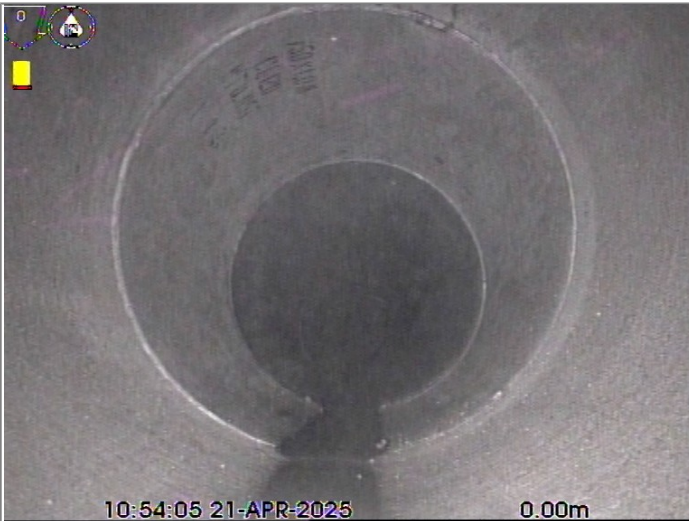
Start node type, manhole, reference S8
