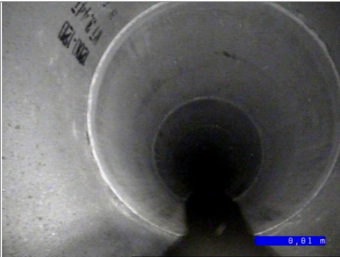
Start node type, manhole, reference SHB3
