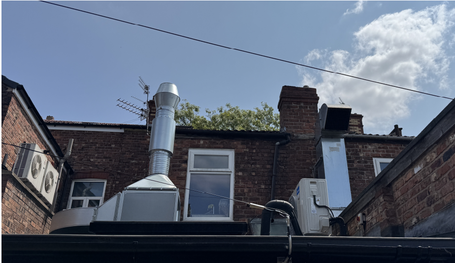
Figure 3. Rear view of property showing flue and A/C
