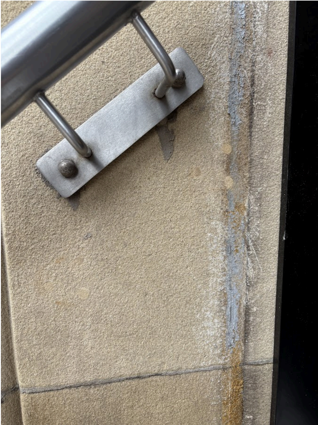
Figure 3.0 - Old handrail holes with colour match sample mortar repair
