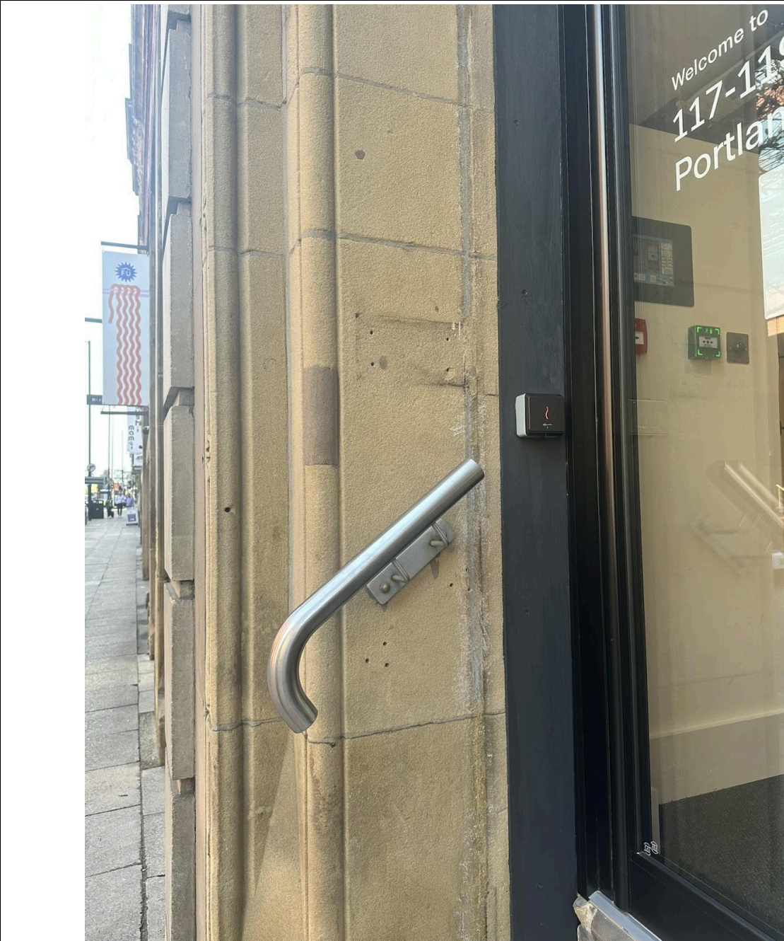
Figure 1.0 - Existing holes for previous sign and handrail
