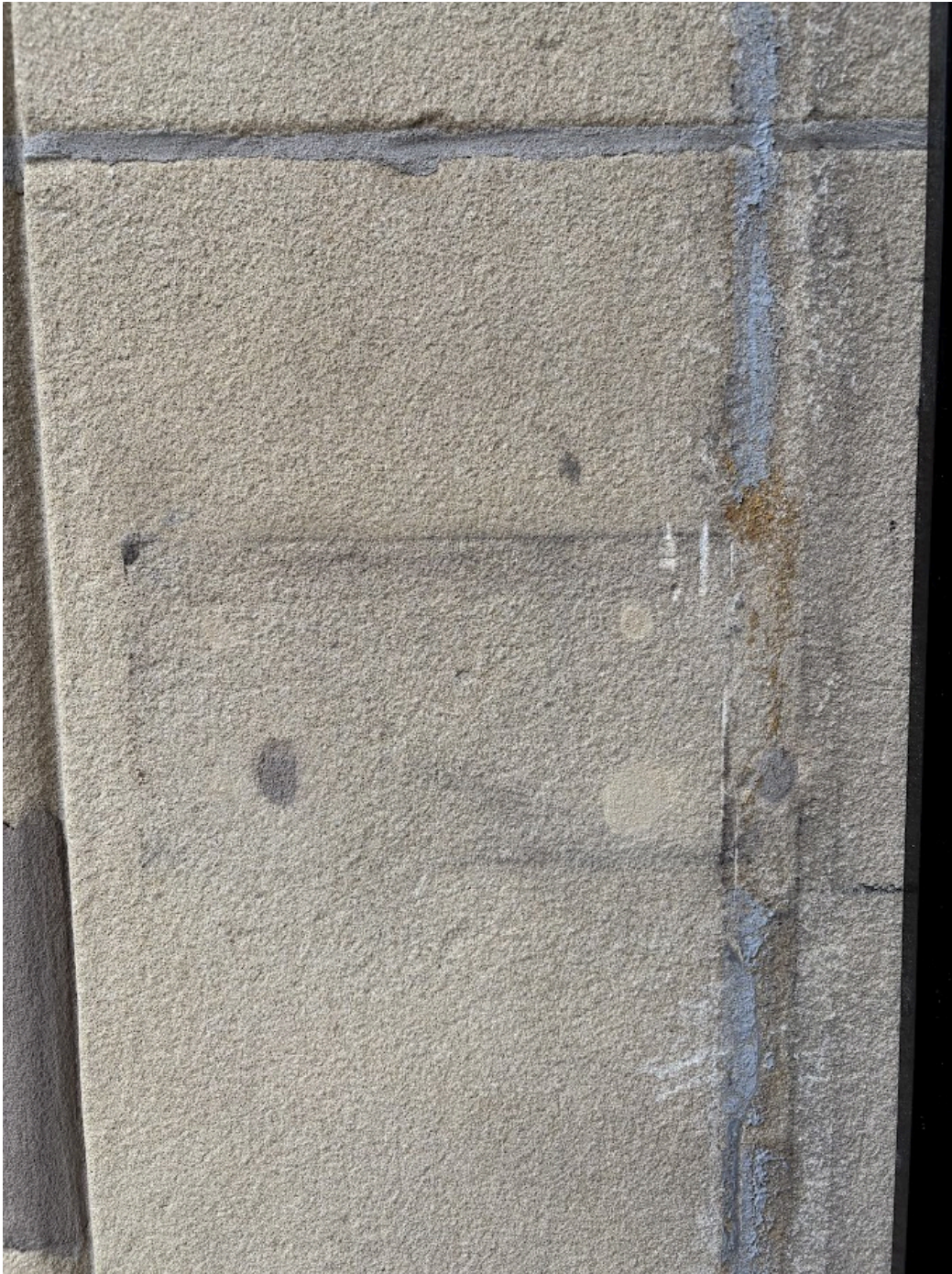
Figure 2.0 - Sign holes repaired with colour match sample mortar repair
