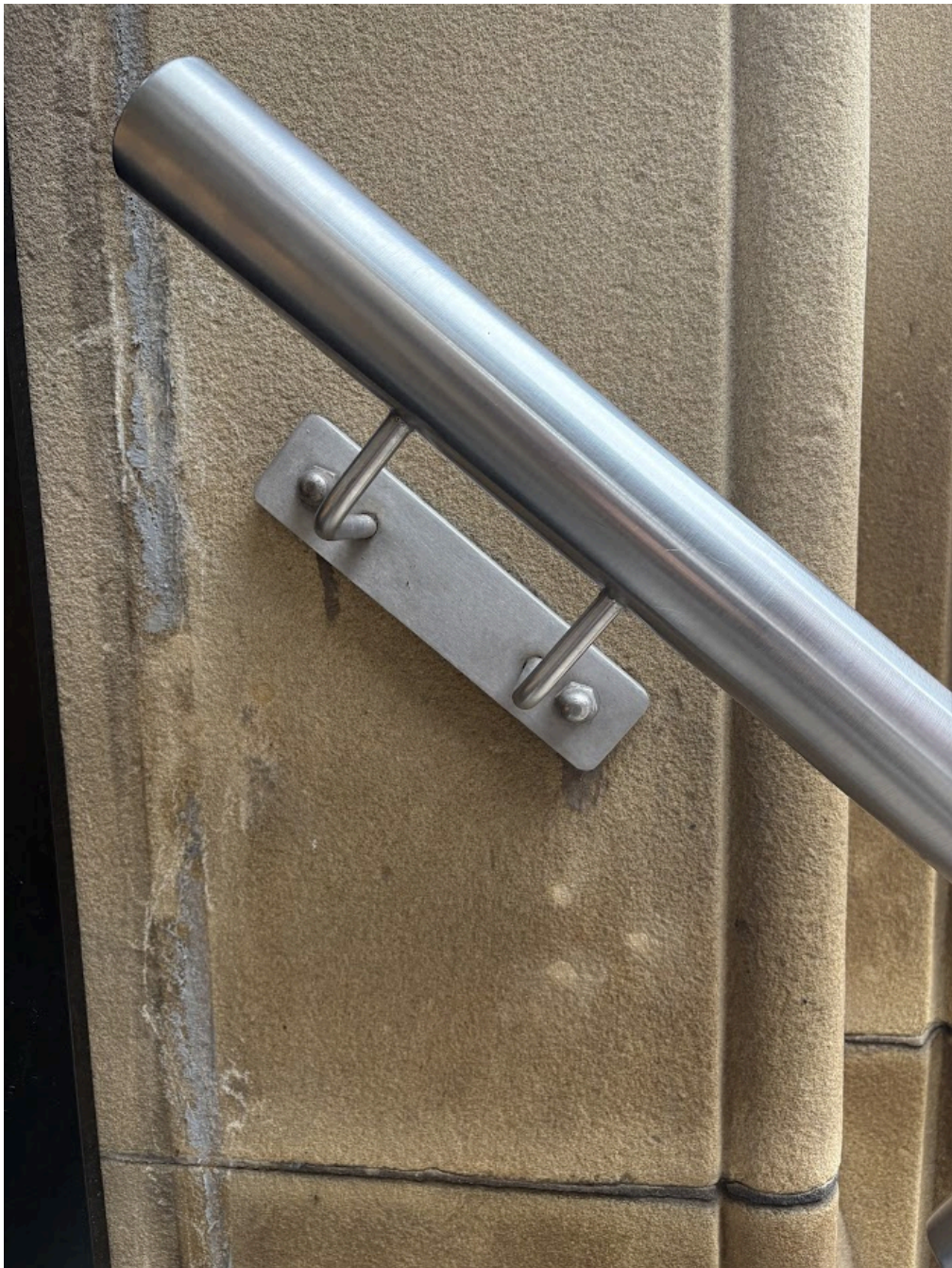
Figure 5.0 - Old handrail holes with colour match sample mortar repair
