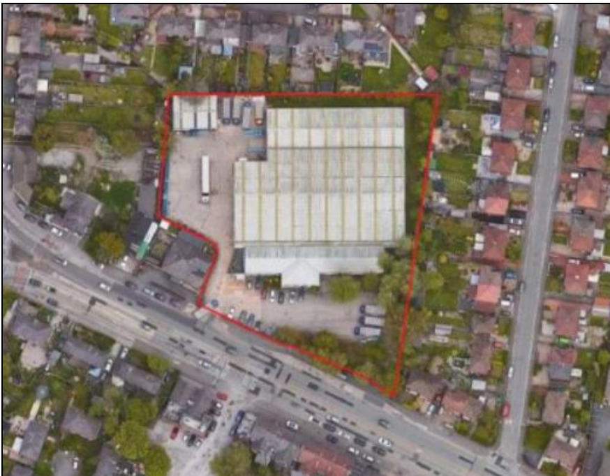
Aerial view of existing site (extract: Design and Access Statement)
