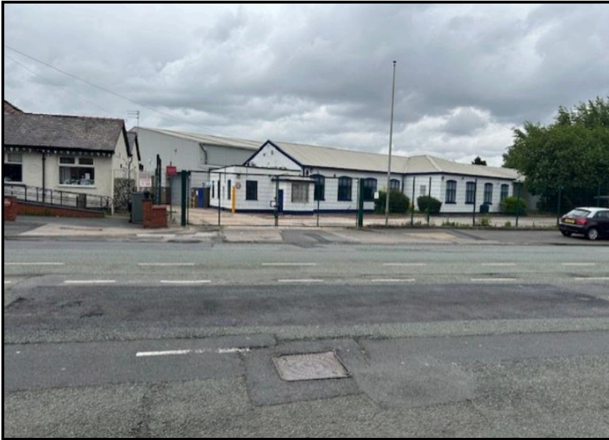
View of application site from Hollinwood Avenue
