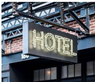
External Tenant Flag Signage Suspended external signage from canopy
