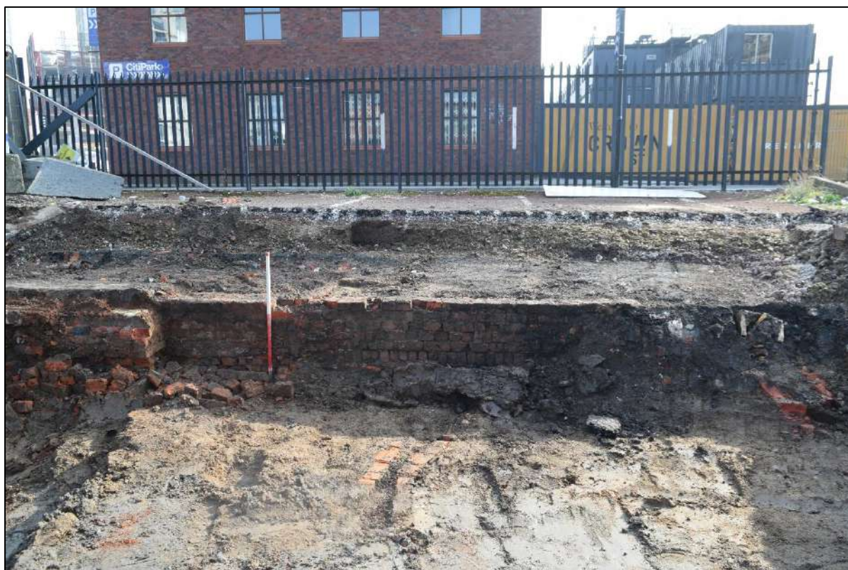
Plate 8: Wall foundation [015] spanning south-east end of Area A, adjacent to Silvercroft Street
