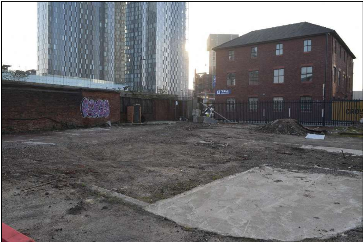
Plate 6: Pre-excavation shot of Area A, looking toward east corner of Site at junction of Great Jackson Street and Silvercroft Street
