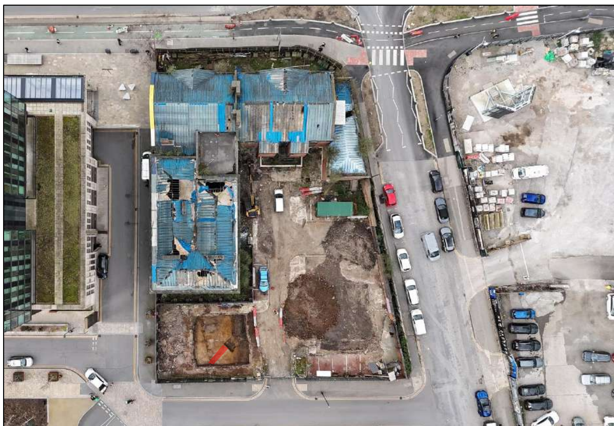
Plate 26: Post-excavation aerial UAV of Bridgewater House with Roman gully [114] indicated.
