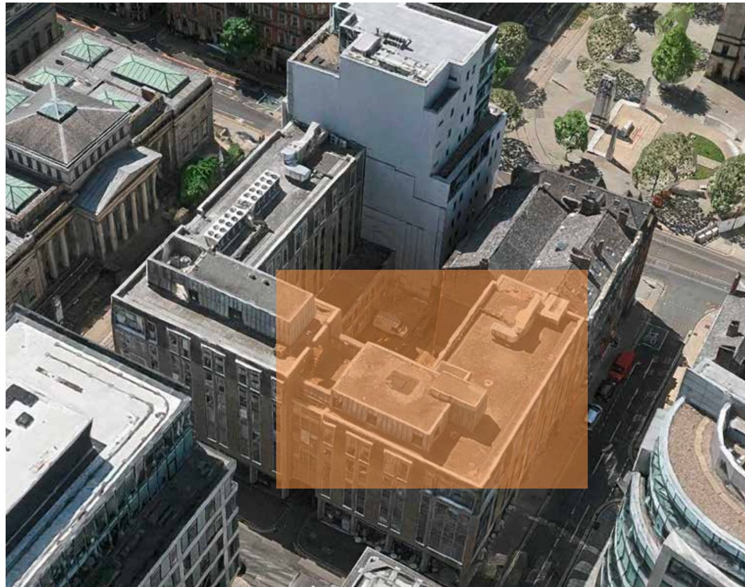
Image: Aerial view of Abbey House with rooftop site highlighted.
