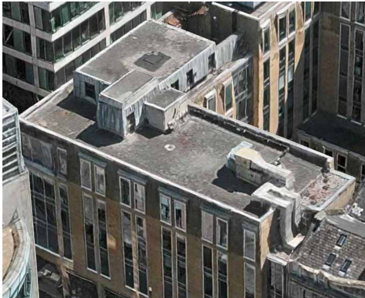
Image: Aerial view of Abbey House as existing.
